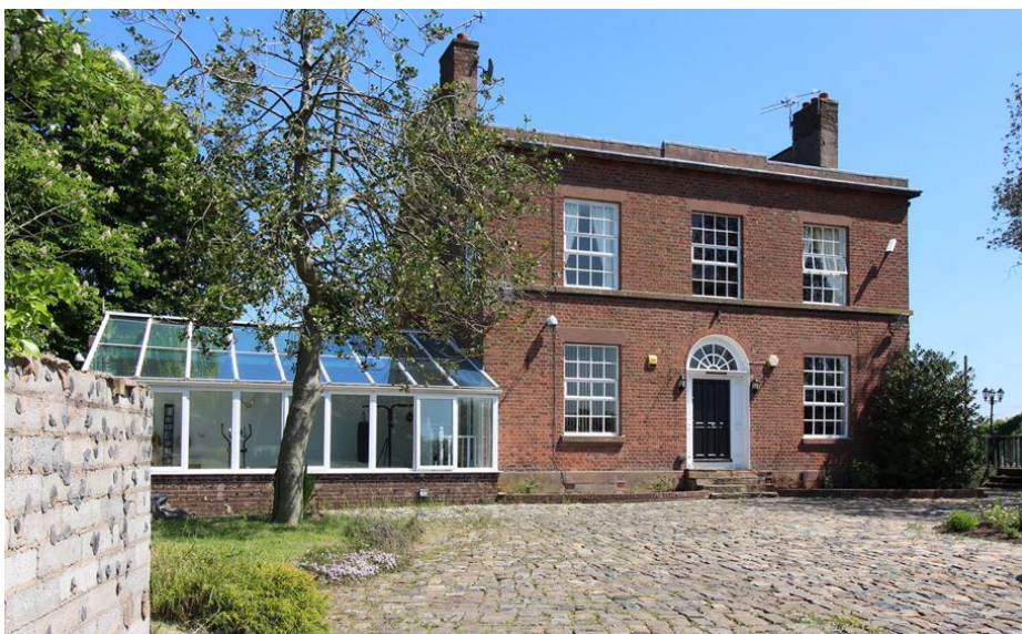
Figure 2: Image showing the front of the property
