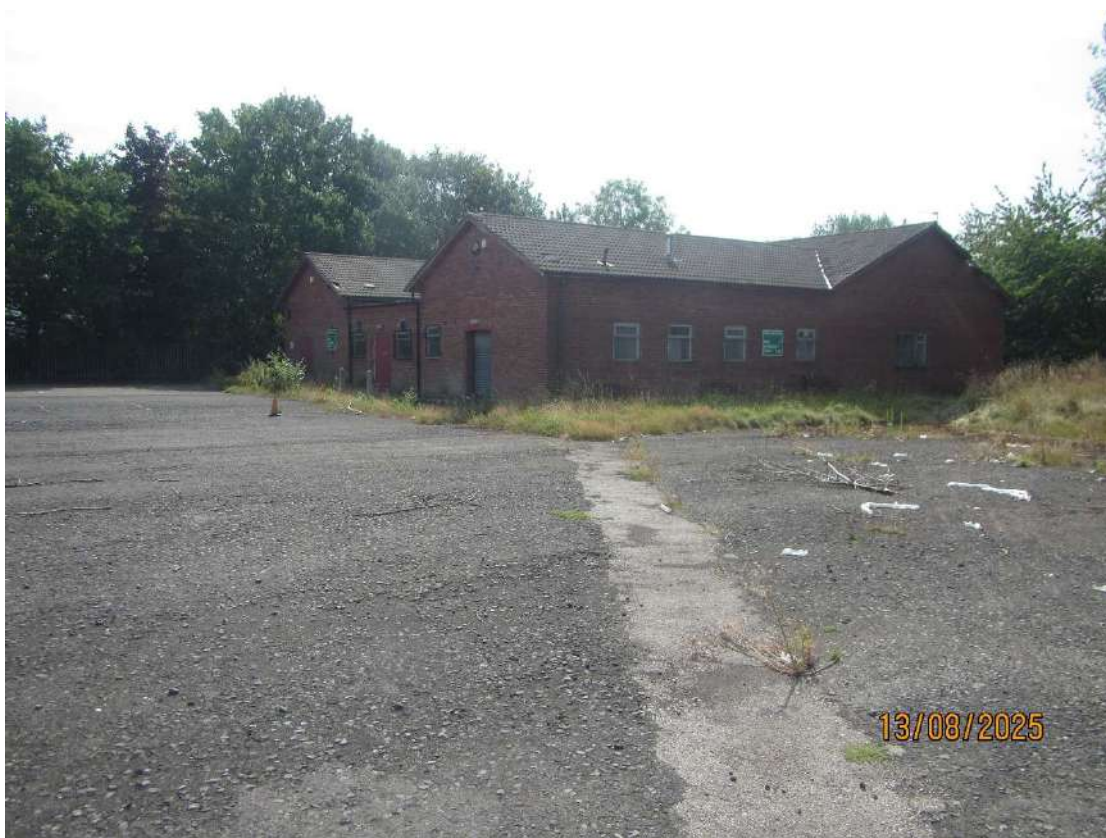
Photograph 12. The northern and western aspects of Building 7.
