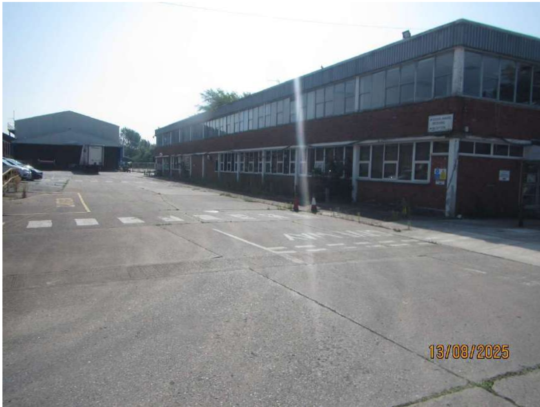
Photograph 7. The northern aspect of Building 2.
