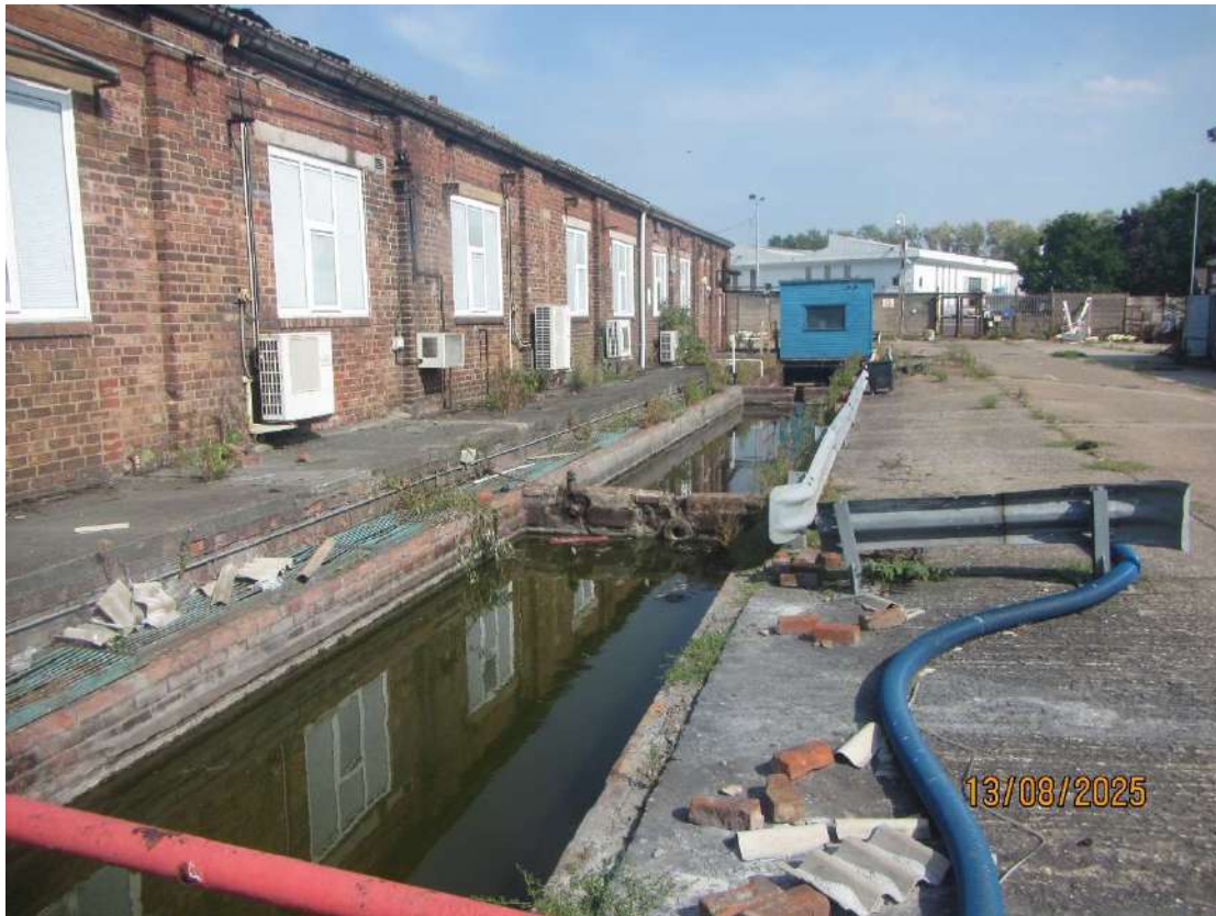
Photograph 3. An industrial lagoon located to the south of Building 1.
