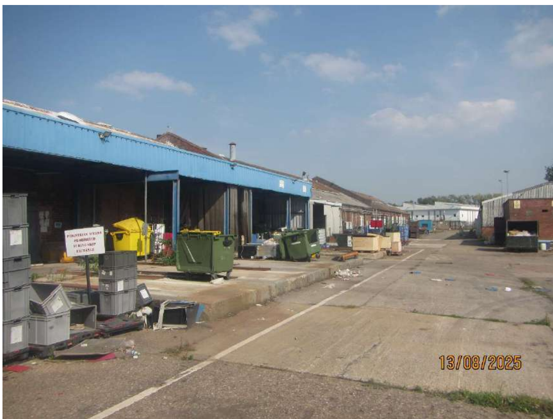
Photograph 4. The southern aspect of Building 1.
