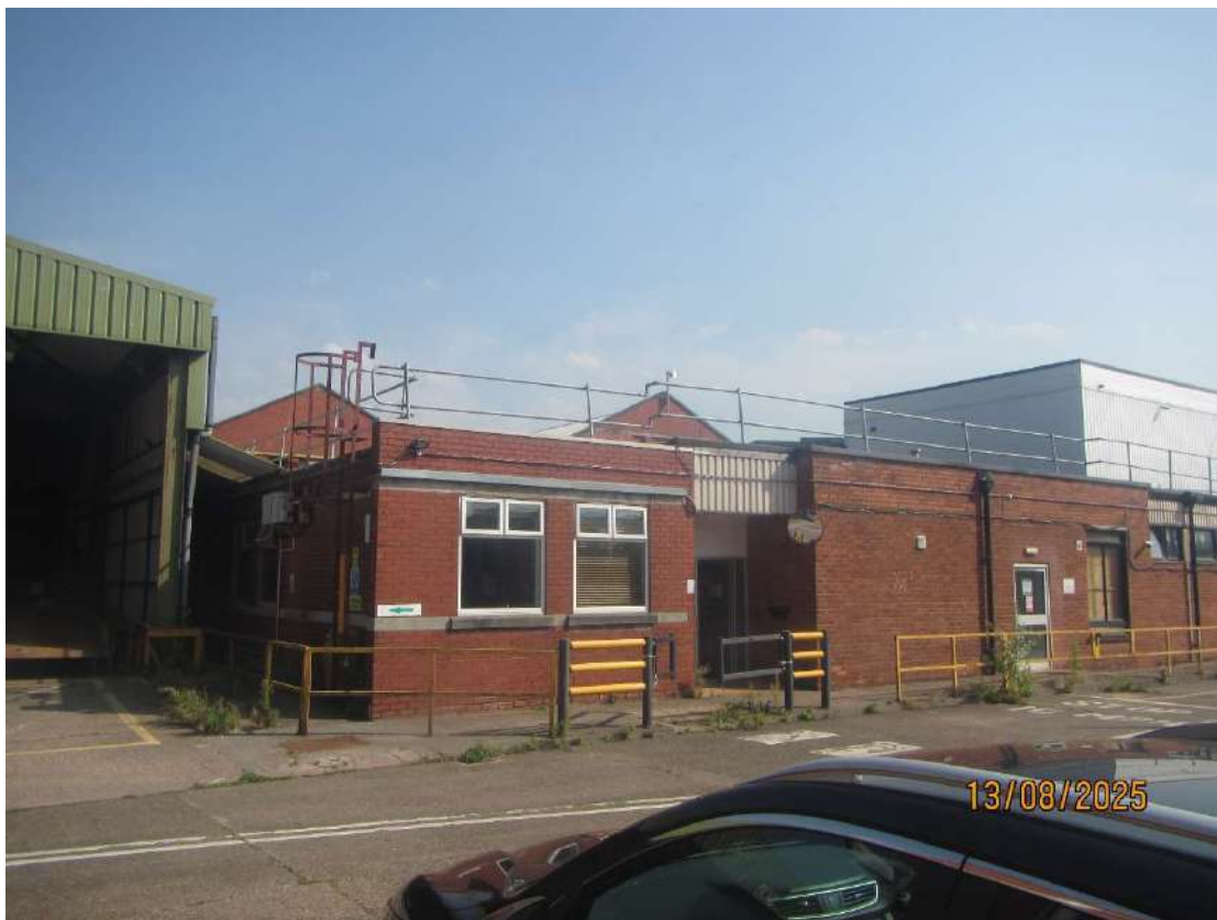
Photograph 5. The western aspect of Building 1.
