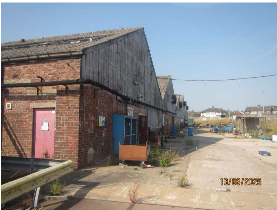
Photograph 6. The eastern aspect of Building 1.
