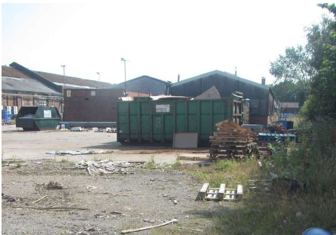
Photograph 8. The western aspect of Building 3.
