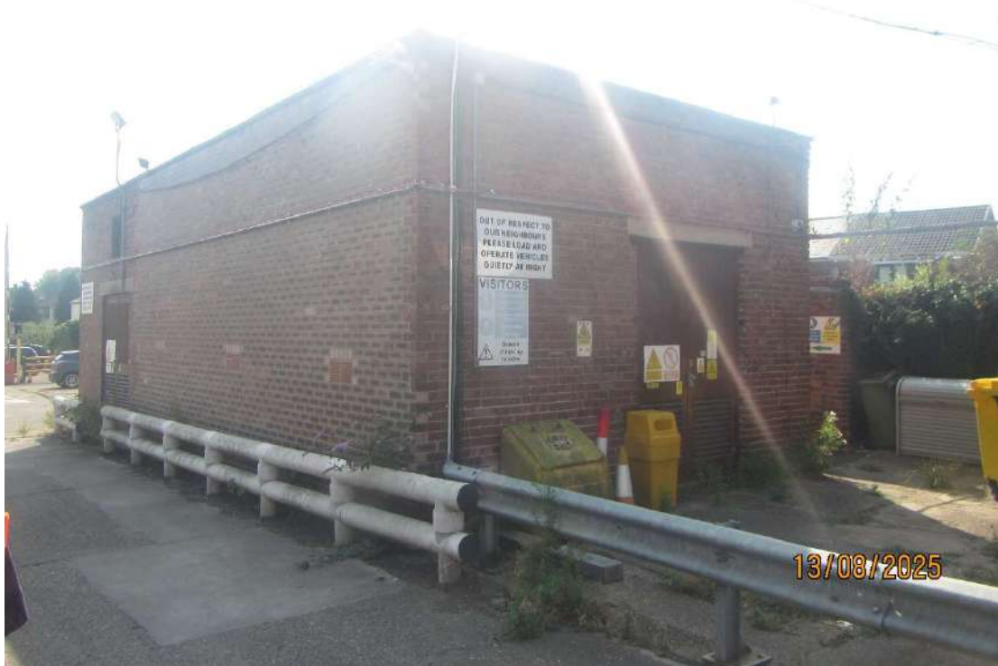
Photograph 11. The northern and eastern aspects of Building 5.
