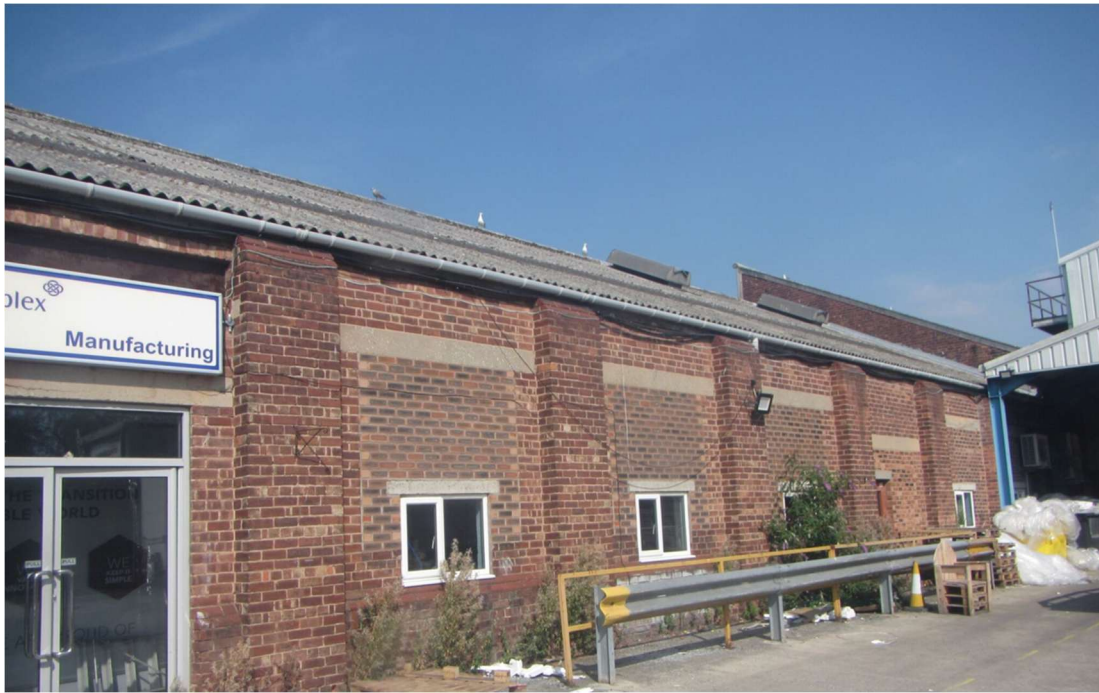
Photograph 3 – Corrugated asbestos roof on Building 1.
