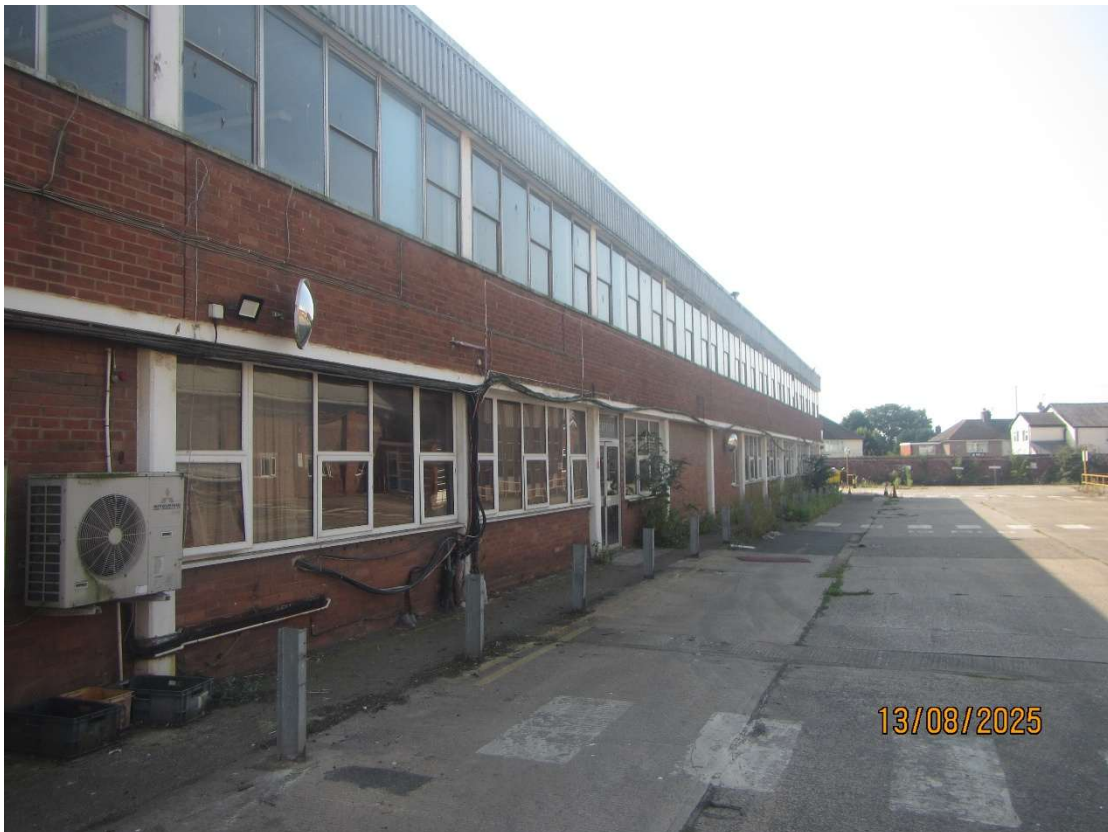
Photograph 10 – The northern aspect of Building 2.
