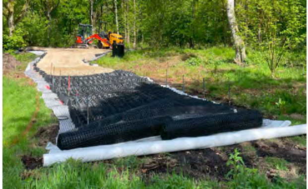
Example of temporary and permanent ground protection systems such as CellwebTRP
