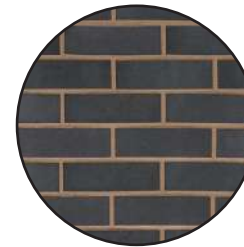
DPC Course Such as Smooth Blue Engineering
