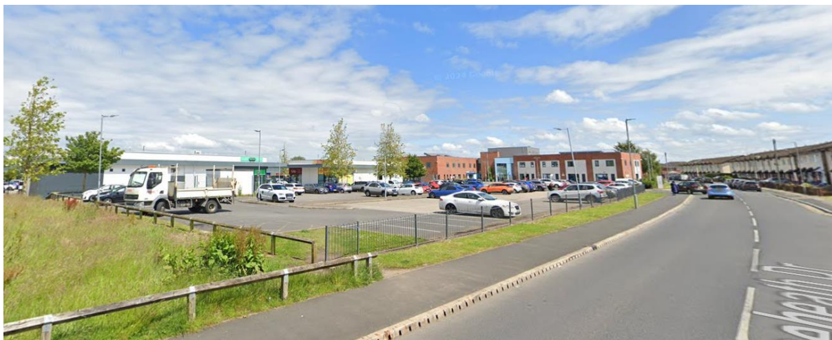
Figure 1. Street view of the application site (Source: Google)
