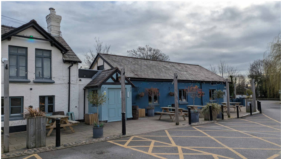
5. Front Elevation - Entrance and Hall
