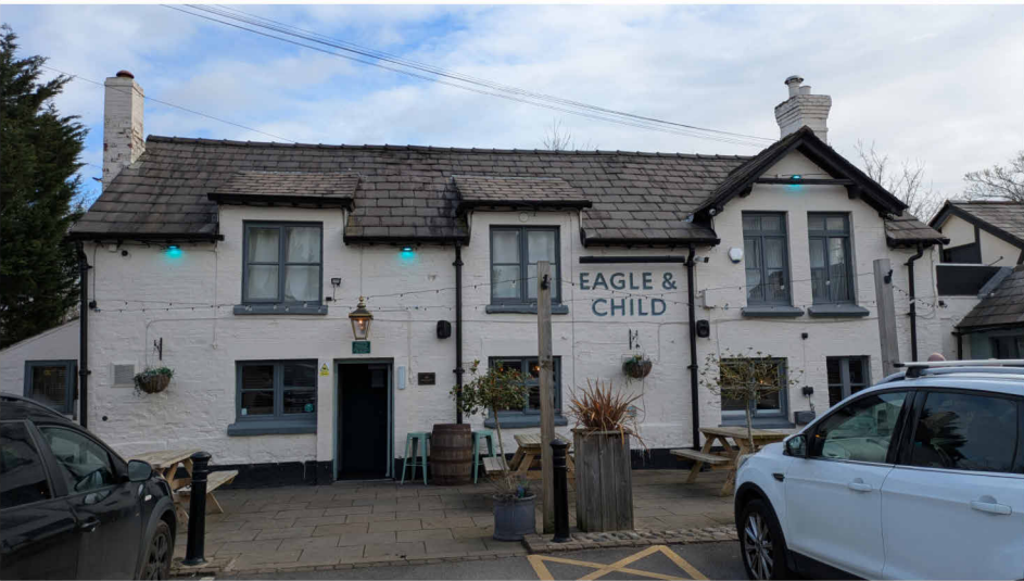
3. Front Elevation - Main Building
