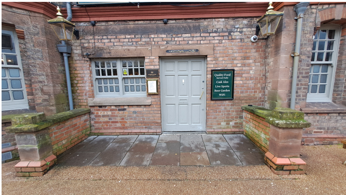
Front main entrance
