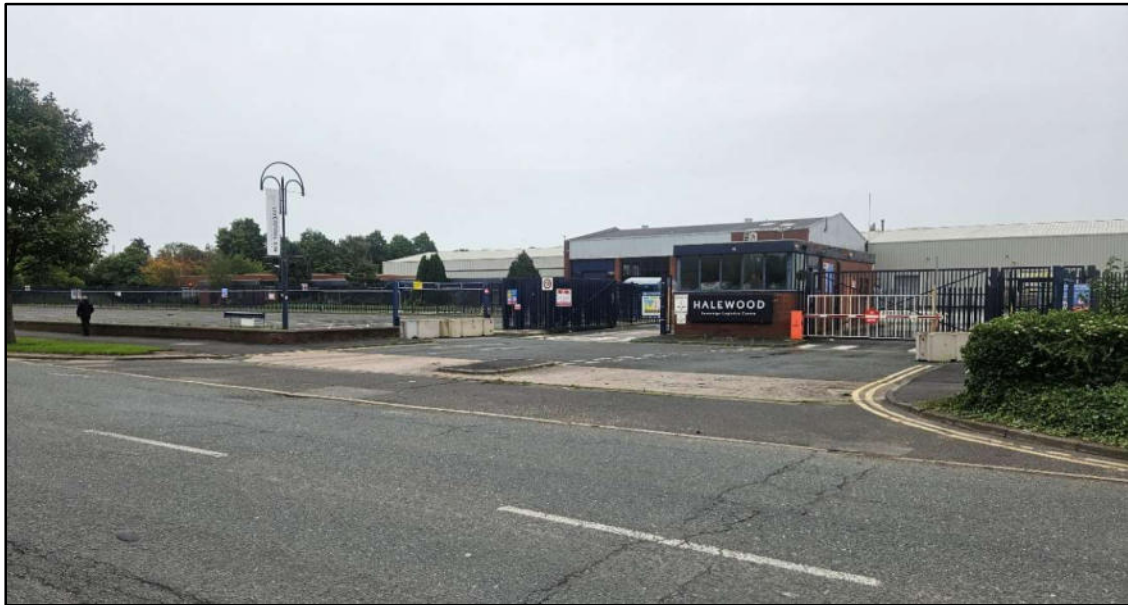
Figure 1.3 Photograph of Existing Industrial Access and Gatehouse with Wilson Road
