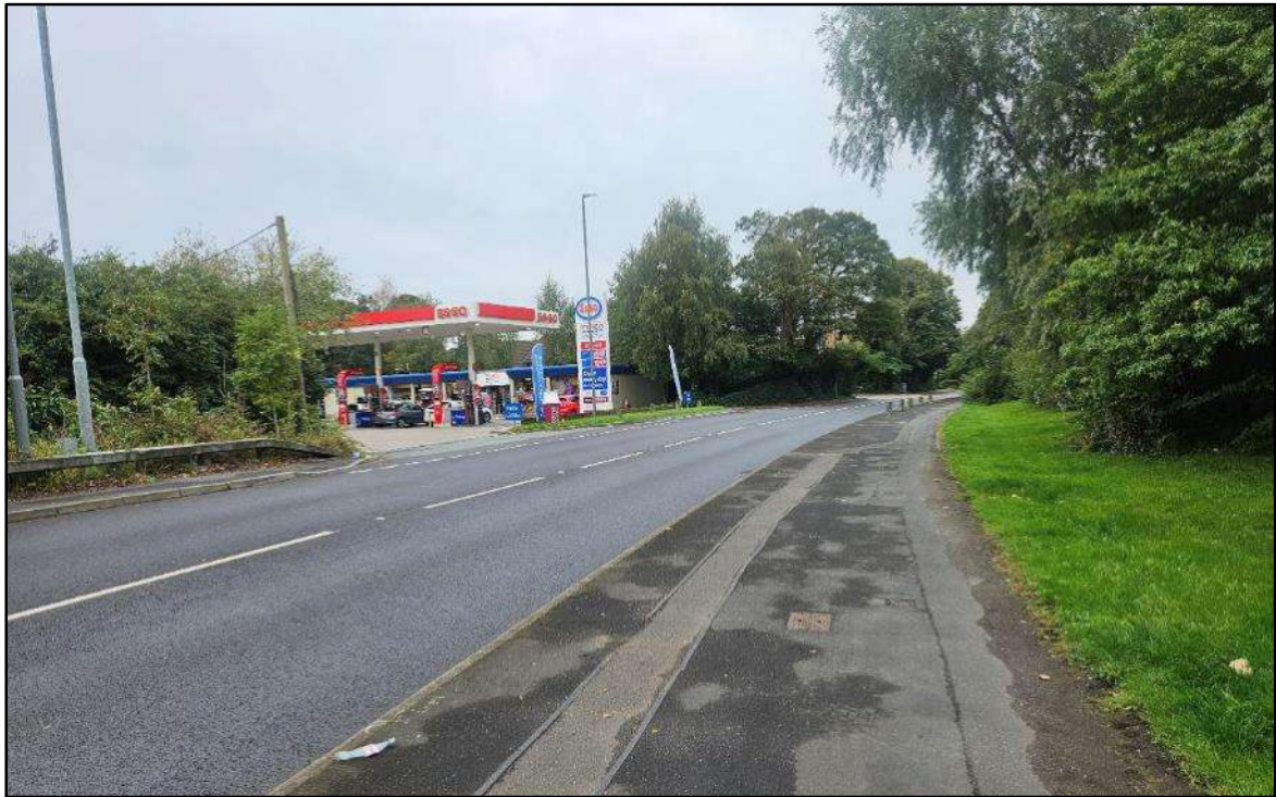
Figure 2.5 Photograph along Cronton Road (looking west)
