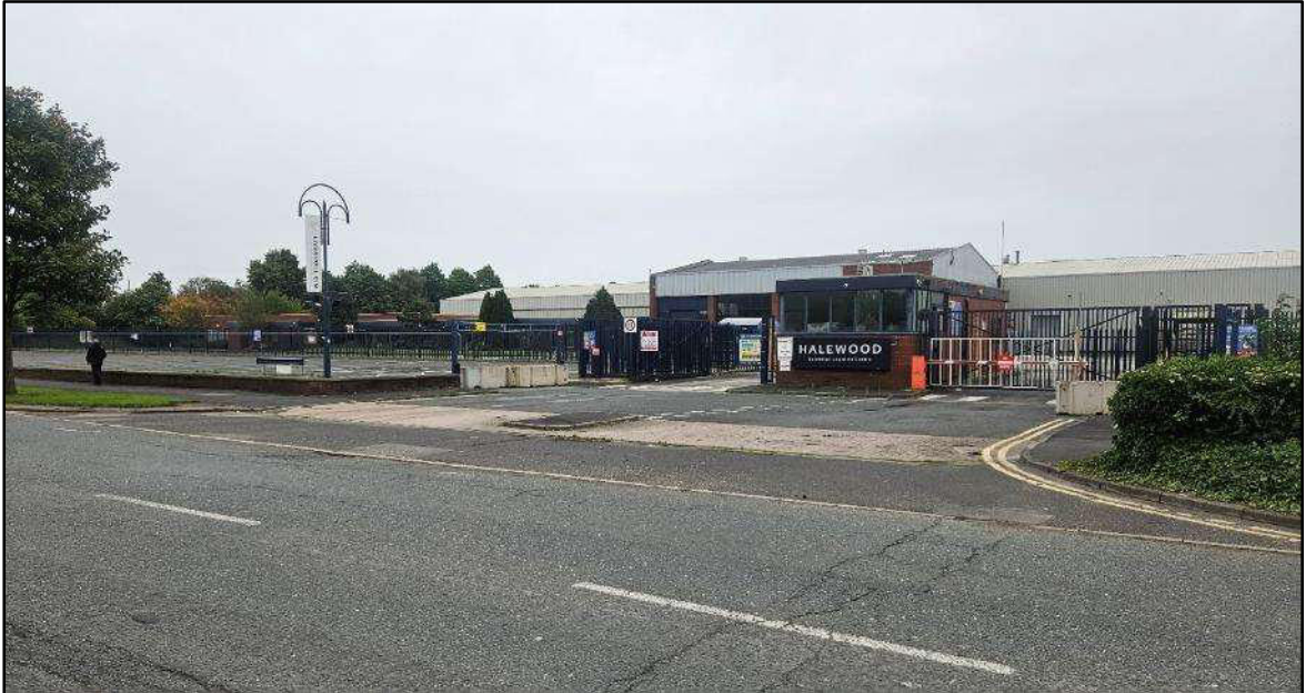
Figure 2.2 Photograph of Existing Industrial Access and Gatehouse with Wilson Road
