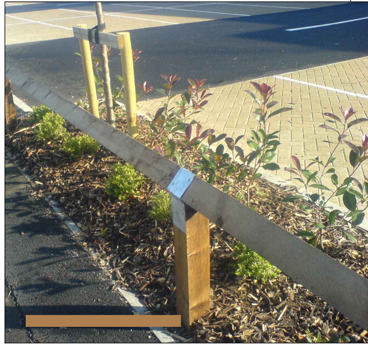
Timber Knee Rail Timber birdsmouth posts, 70 x 70mm, with a top rail 91 x 91mm.
