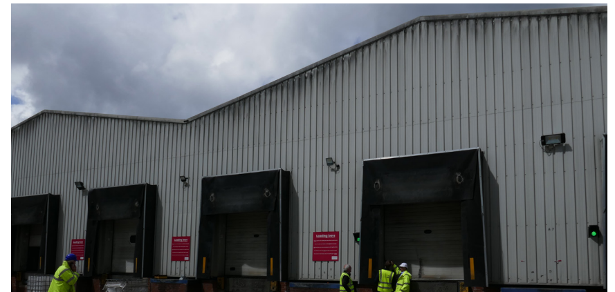
View of the southern elevation of Block A showing dock levellers.
