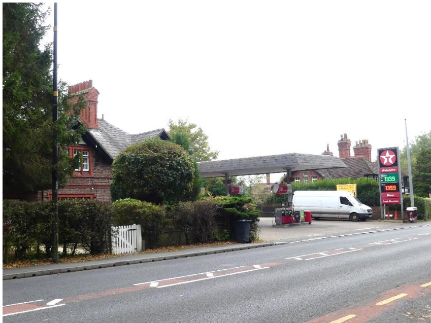
Figure 4.9: The petrol filling station positioned amongst the estate houses, Knowsley Lane
