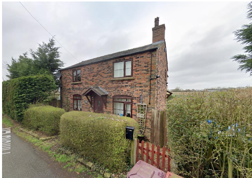
Figure 6 – Views of Pinfold Cottage from Pinfold Lane.
