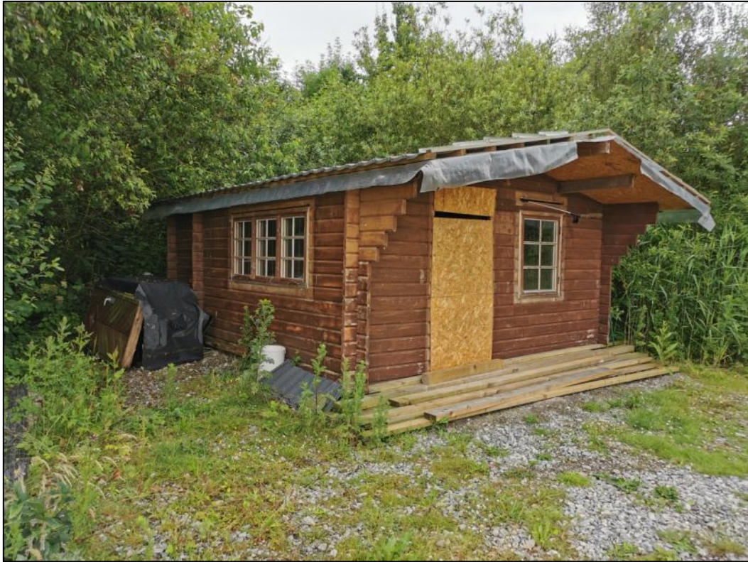
Plate 9 – Hut building, front, north-facing aspect
