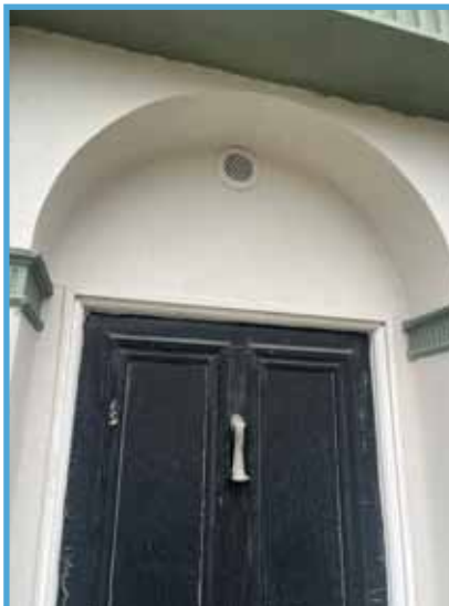
Existing front entrance door head
