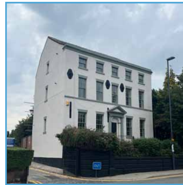
View from High Street
