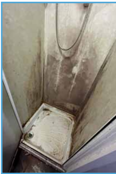
Existing shower to rear of front entrance
