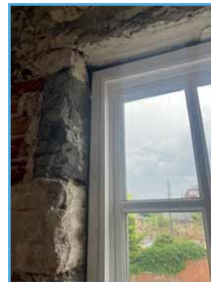
Example of 1980s workmanship to infill window sash with lightweight blockwork
