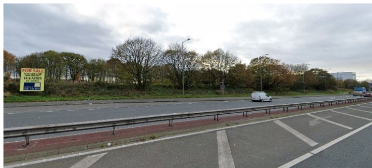
Site Photo P2 – East Lancashire Road toward the development site
