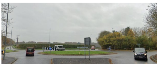
Site Photo P6 – Knowsley Lane & Ormskirk Road roundabout
