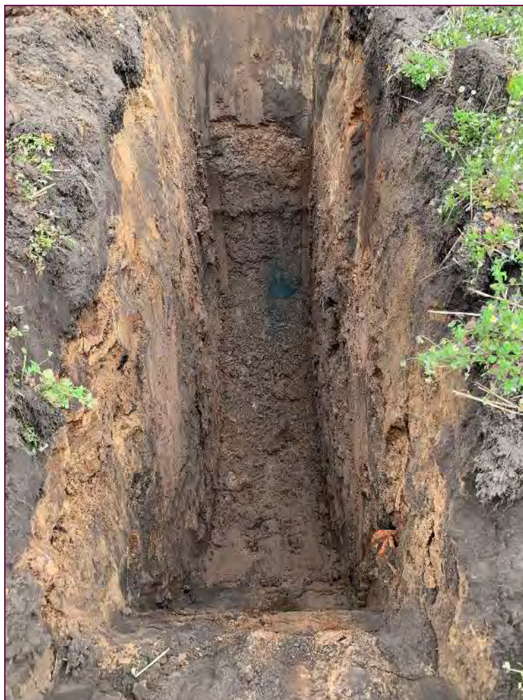
Photograph 6: View of TP105.
