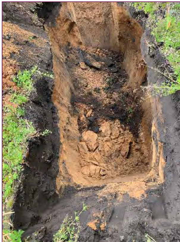
Photograph 7: A view of the side walls collapsing in TP115.
