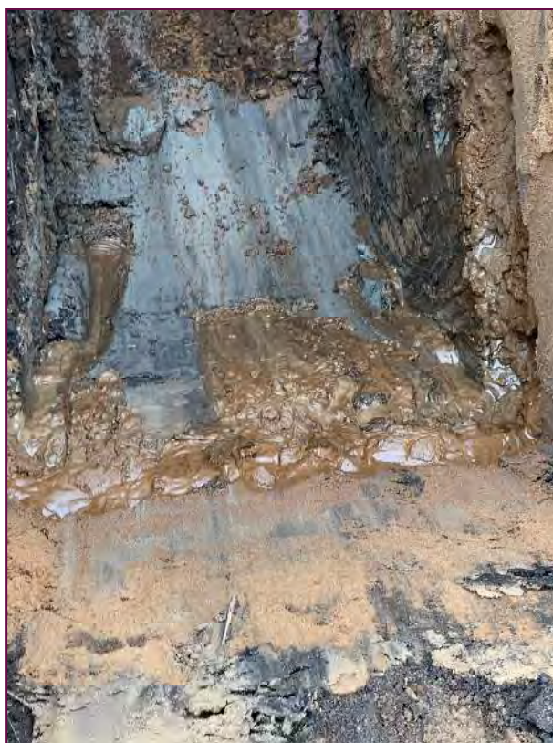
Photograph 8: A view of the running sand (within sand lenses) in TP119.
