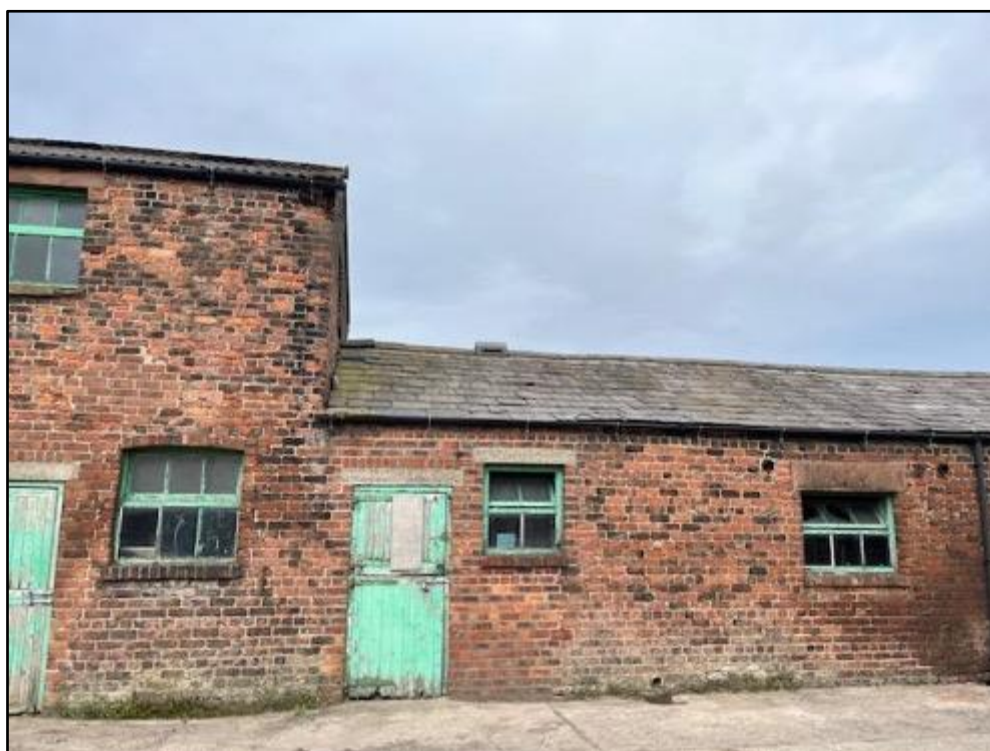
Fig 5: A view of the slate roof section of the building.
