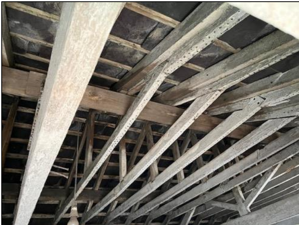
Fig 9: A view of the internal roof space within the northern section of the barn. Wooden beams and rafters sit beneath the slate tiles. No deep cavities were noted within the external walls; there is also a lack of obvious crawlspace or areas suitable for roosting bats.
