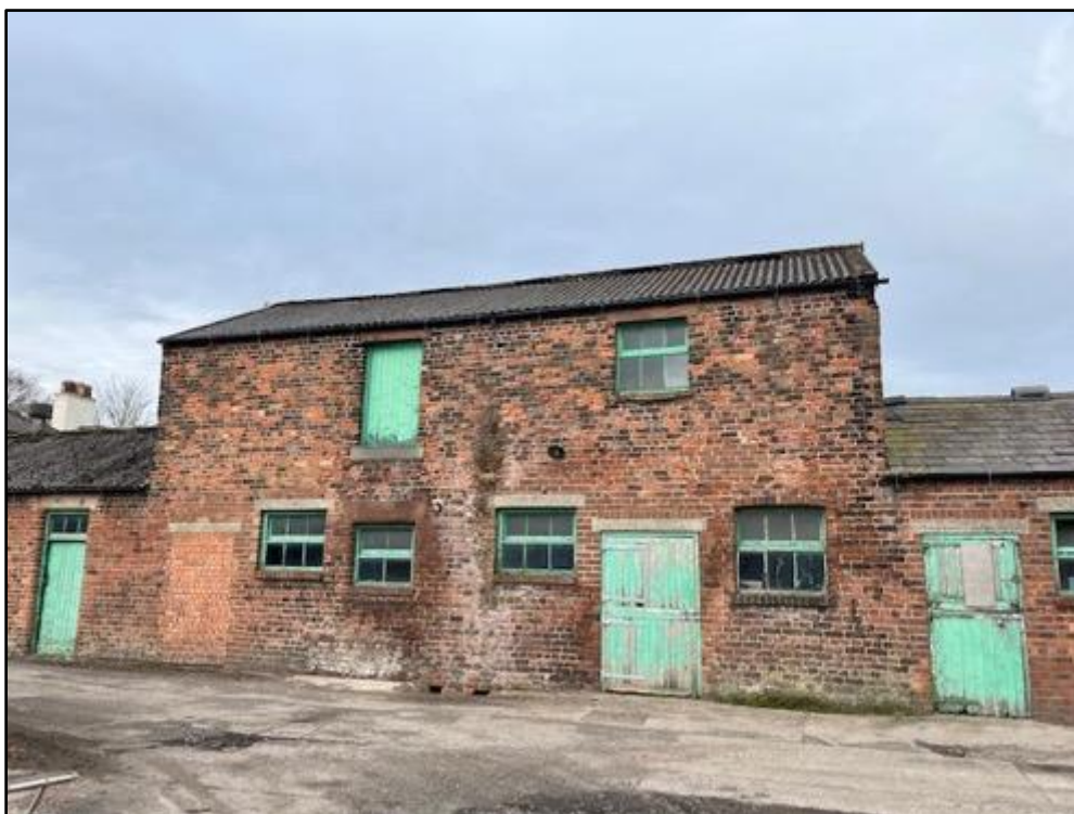
Fig 4: A view of the subject building. The middle section of the building is in a two-storey configuration, with a corrugated asbestos roof atop.
