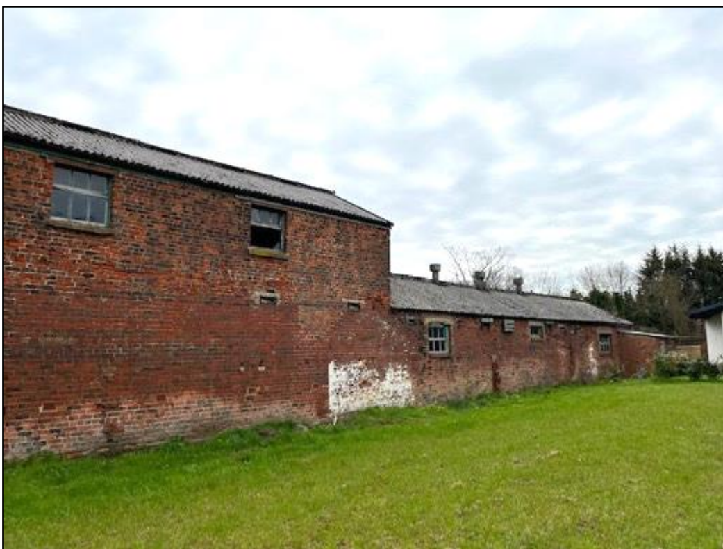
Fig 11: A view from the western side of the building.
