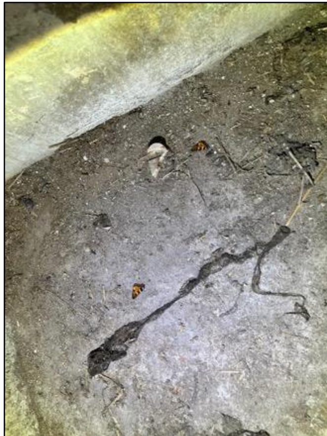
Fig 11: Feeding remains found within the building.
