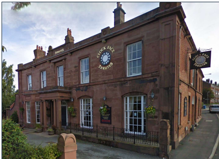
Plate 4 – September 2011: previously installed building mounted first floor sign and amenity board sign to the southwest elevation.
