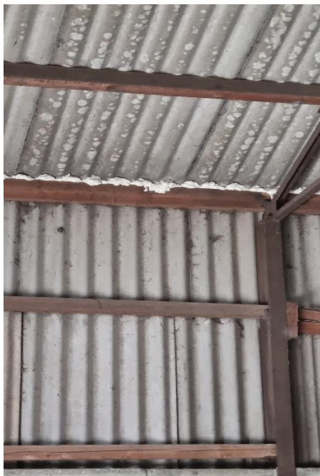
(Foam filler – gaps at the Eaves)
