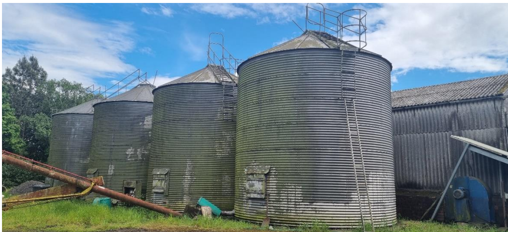
(Unsafe access to monitor moisture content and to load on contract)
