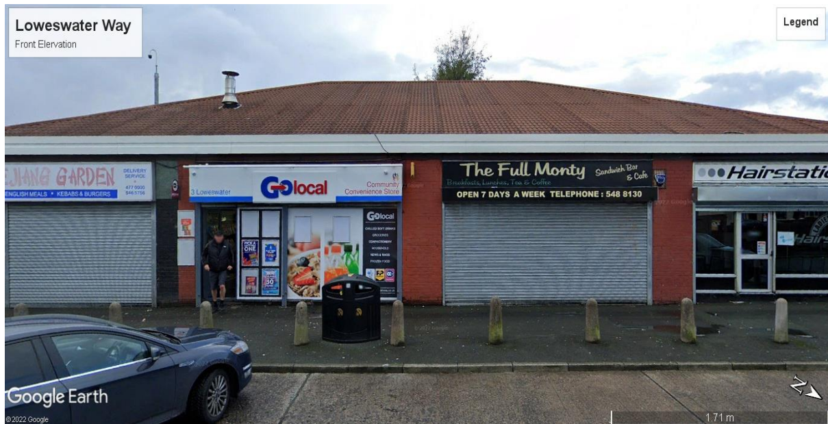
Front elevation of 3-5 Loweswater Way Showing the existing shopfront signage
