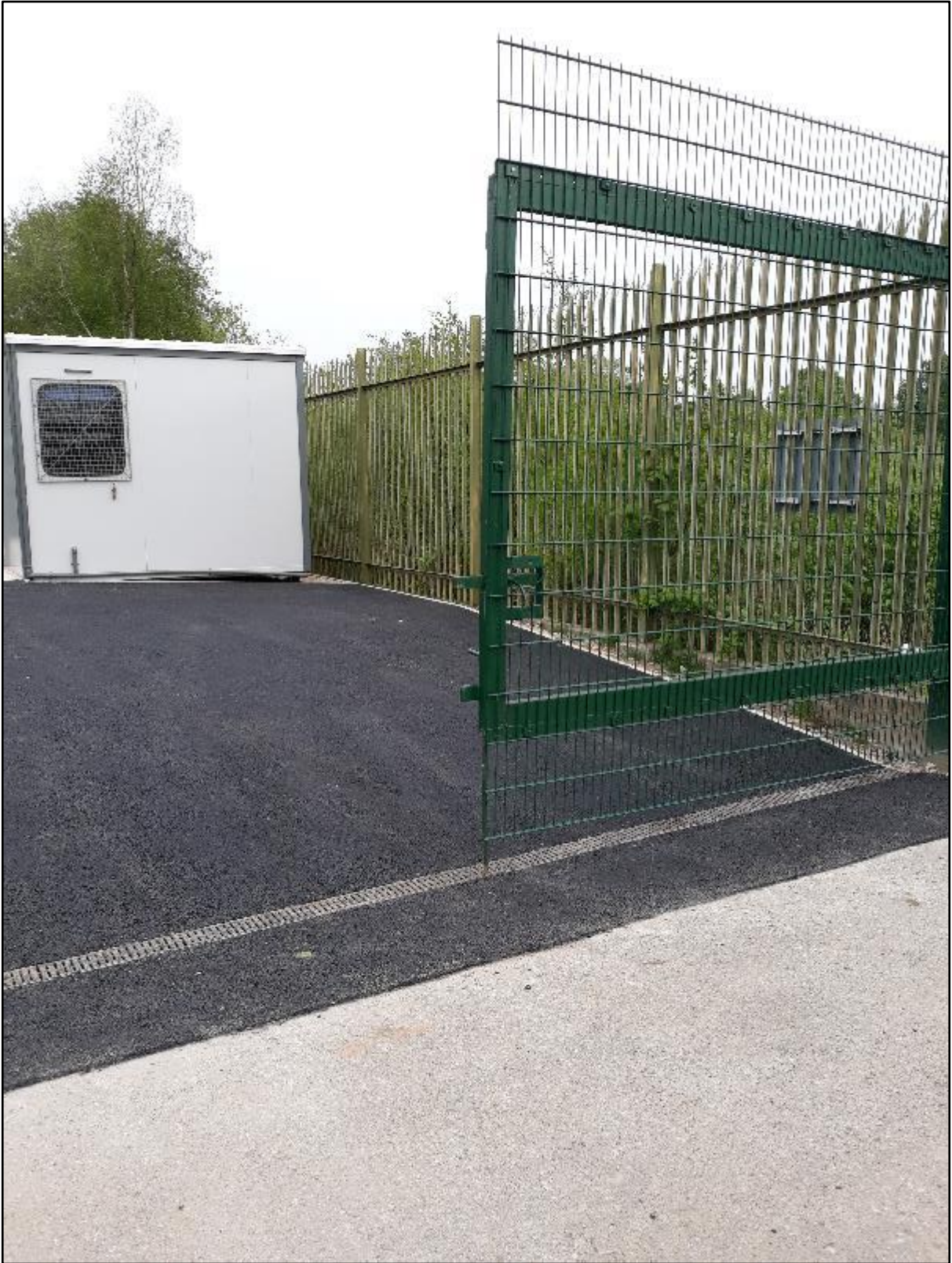
Entrance gate to Backwash area and side elevation Cabin A
