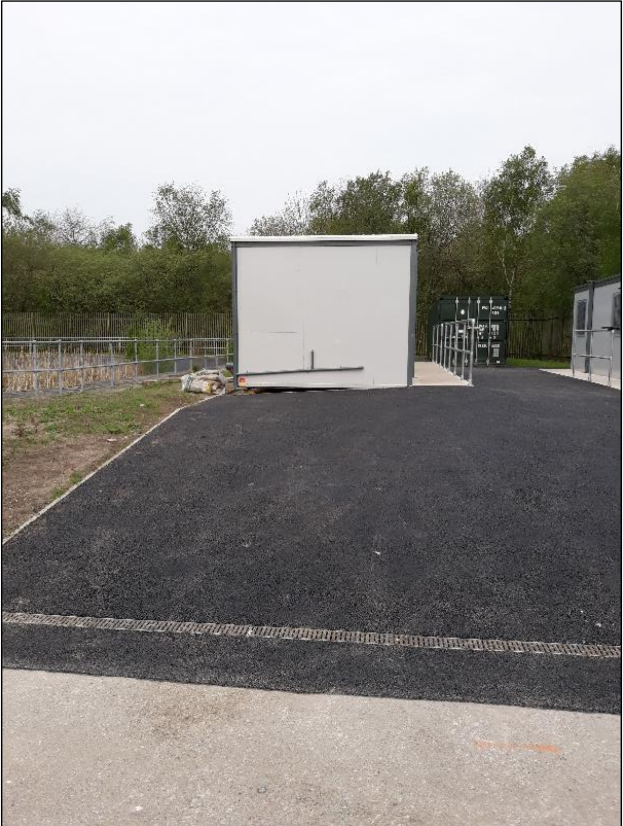
Cabin B&A also showing front of storage container
