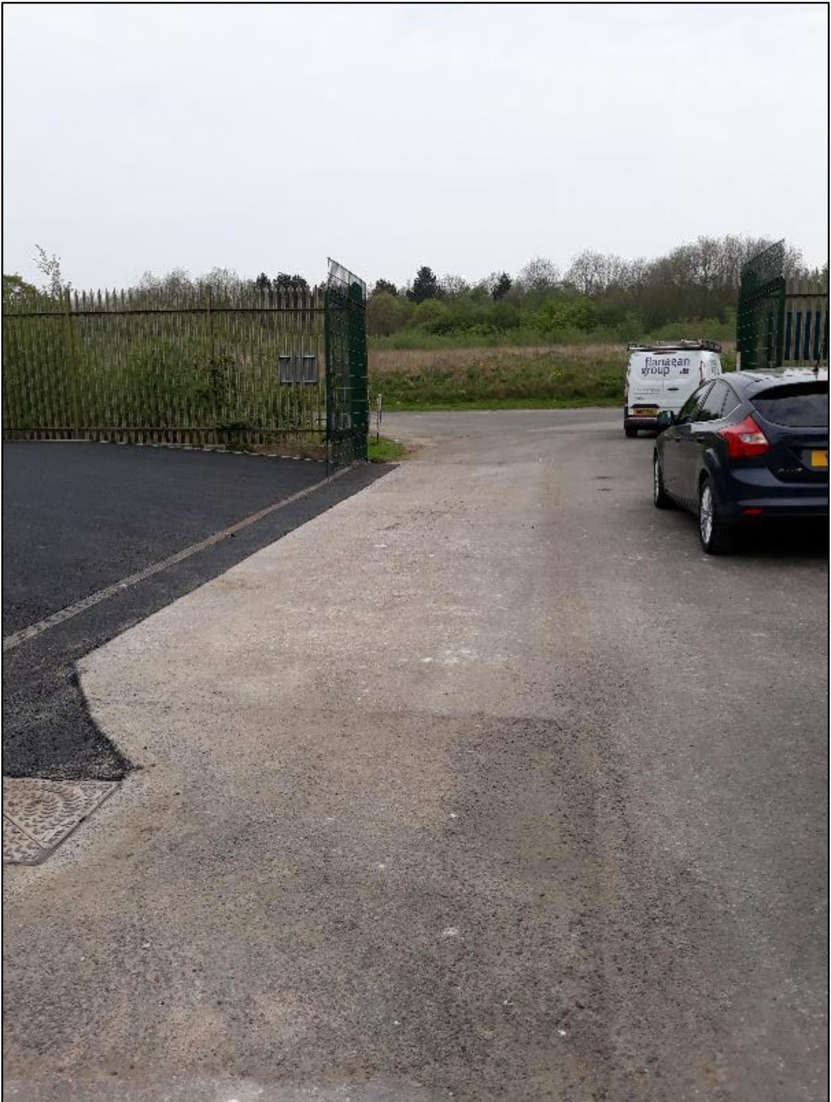
Site entrance gates looking away from site
