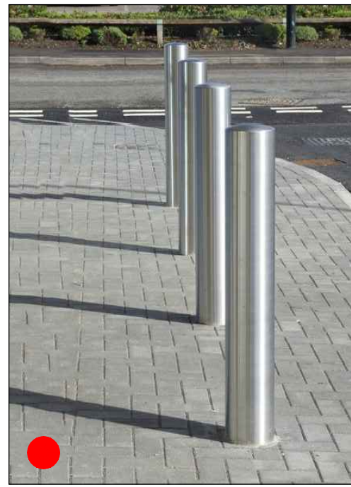
Bollard Type 1 - Impact Protection Steel posts, 1100mm high. Concrete filled, stainless steel. Bolted to concrete hardstand.
