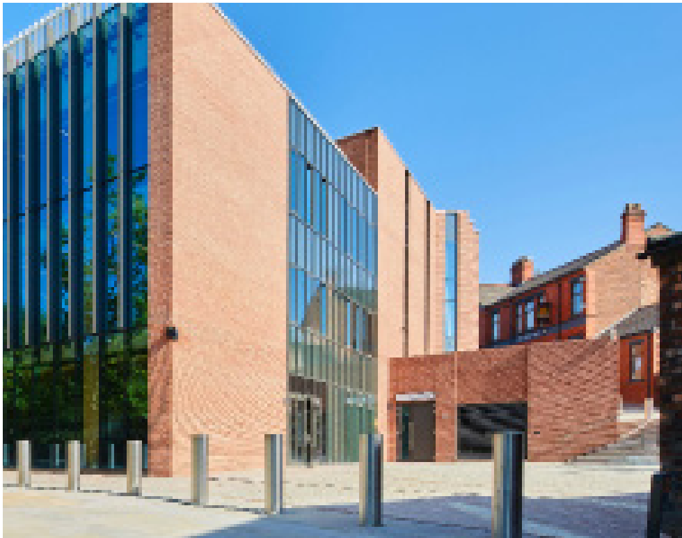
The substation seen from Prospero Place
