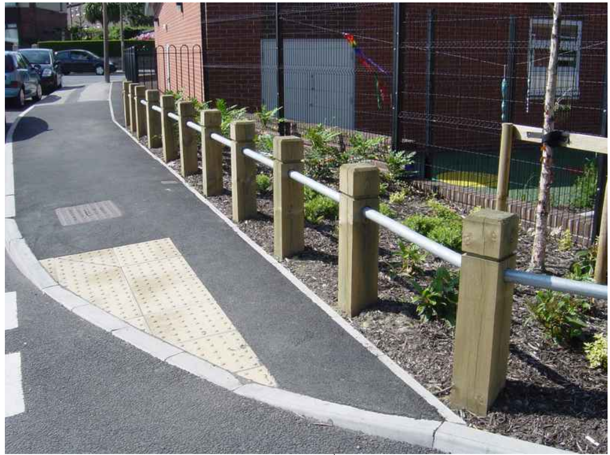
Timber post with metal rail fence.
