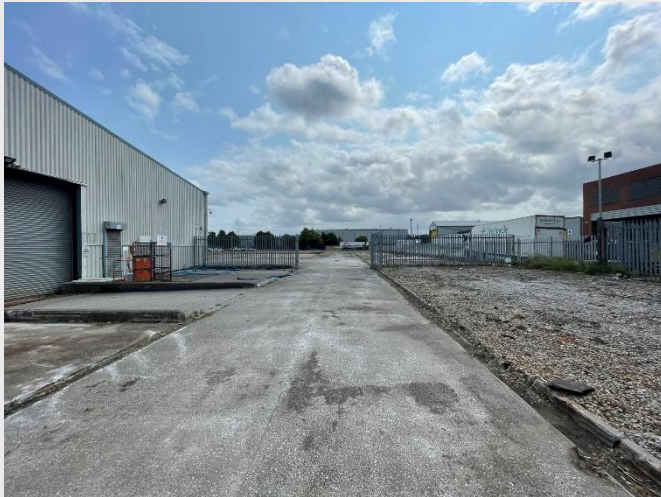
Photograph 11: Combination of habitats onsite, including u1b5, u1b6, u1c and scattered ephemeral and ruderal stands.
