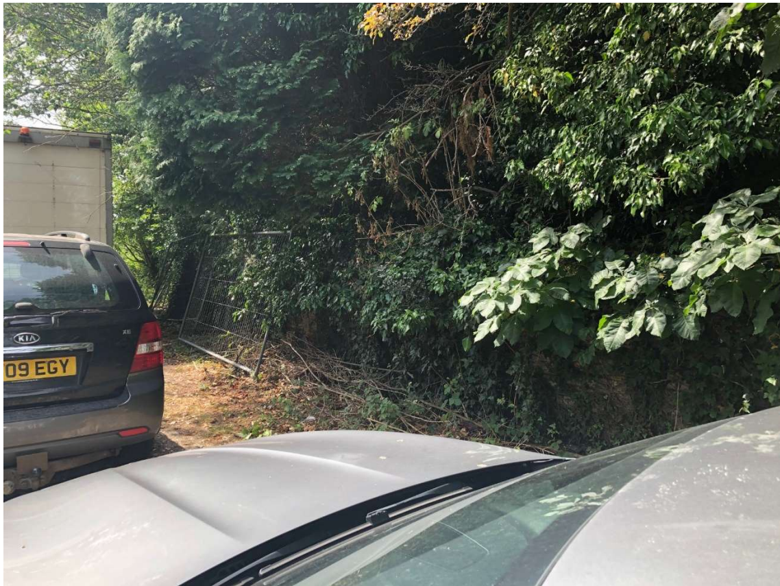
Photo 7 – Photo showing mid section of the wall along the access road. Photos also shows extent of existing vegetation to be removed and existing trees to neighbouring land.
