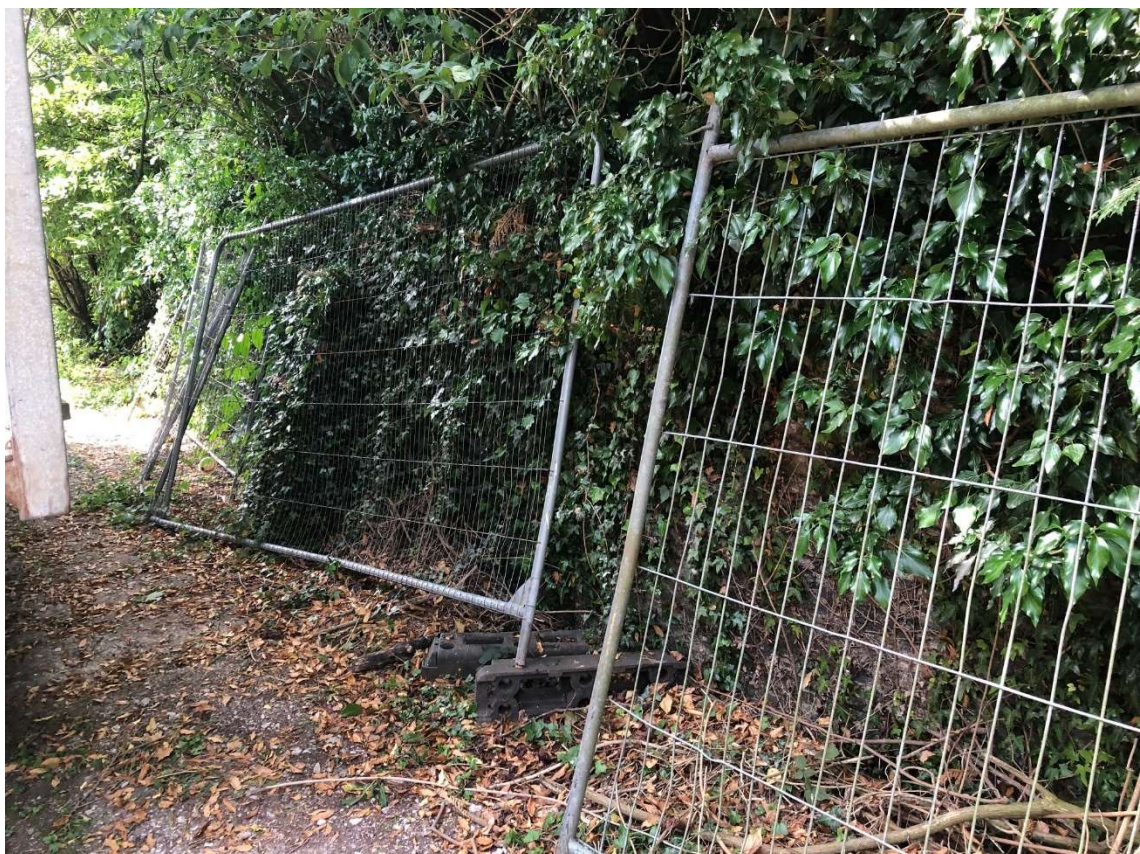
Photo 6 – Photo showing mid section of the wall along the access road
