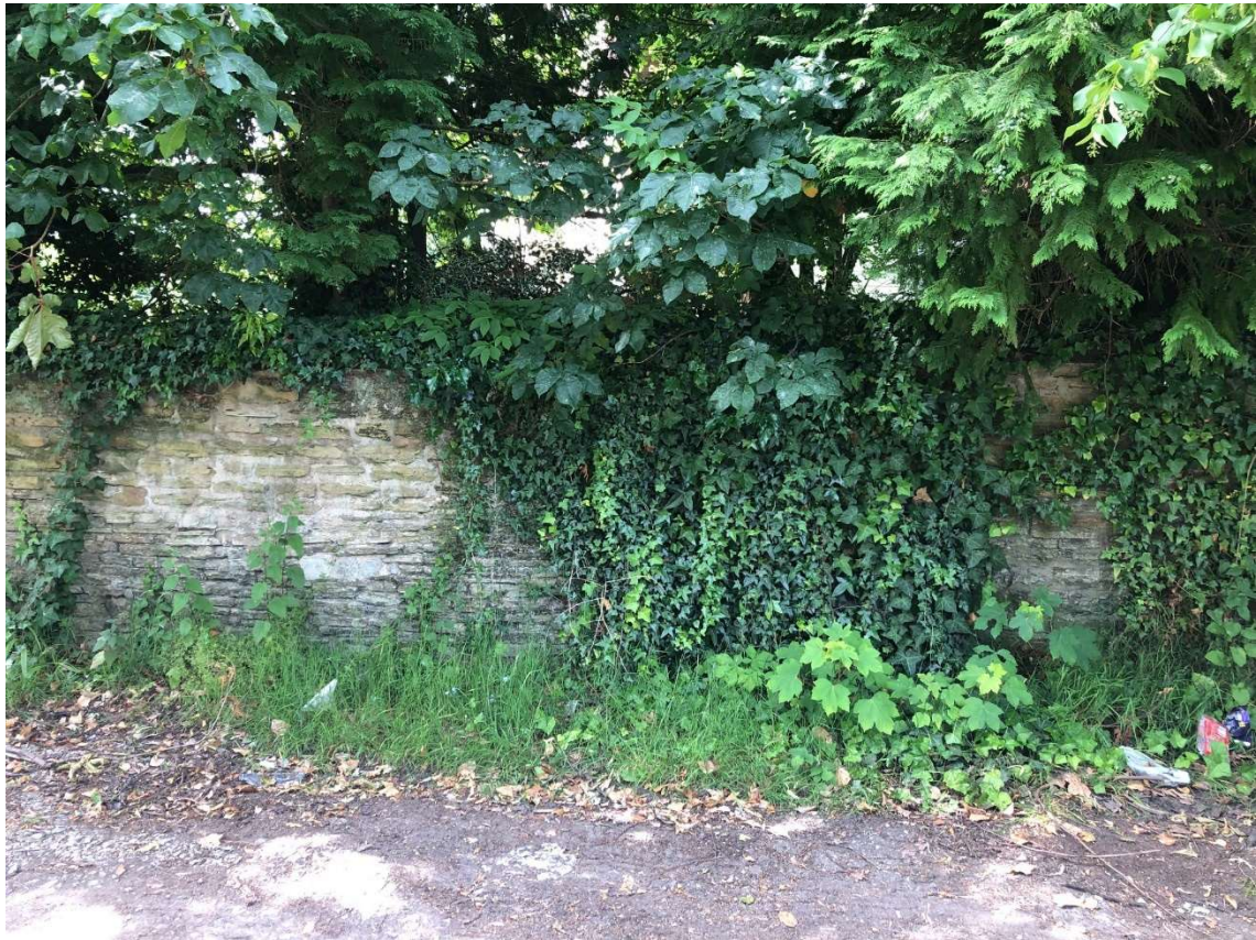
Photo 5 – Photo of the wall at the start of the access road
