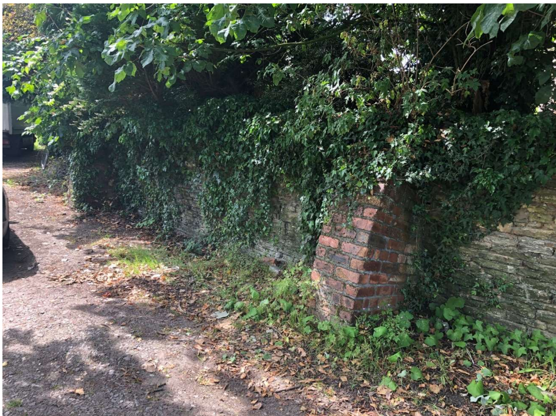
Photo 4 – Photo showing start of access road and brickwork buttresses
