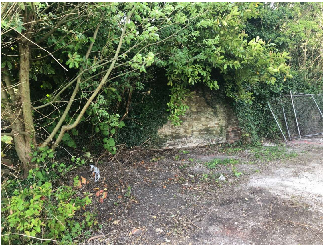
Photo 2 – View of wall at end of access road closest to the development site
