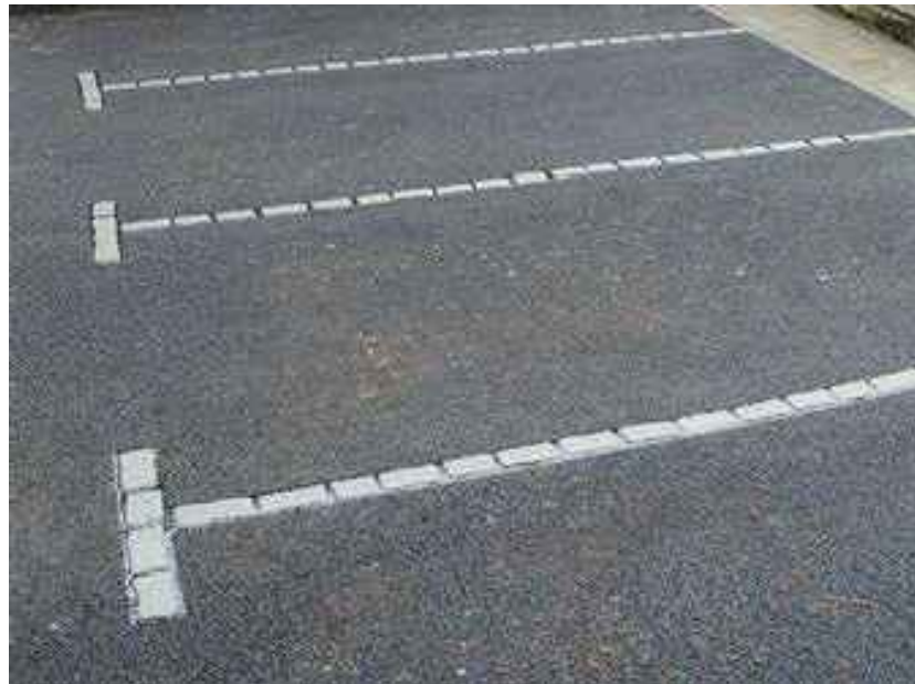
Black Tarmac to Car Park with Stone Sett Markings (4)
