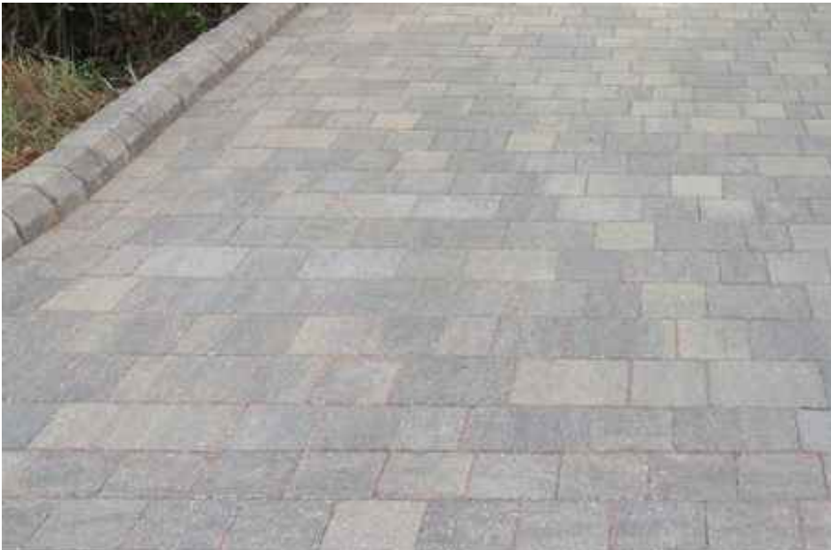
Block Paving / Stone Setts to Access Road (1)
