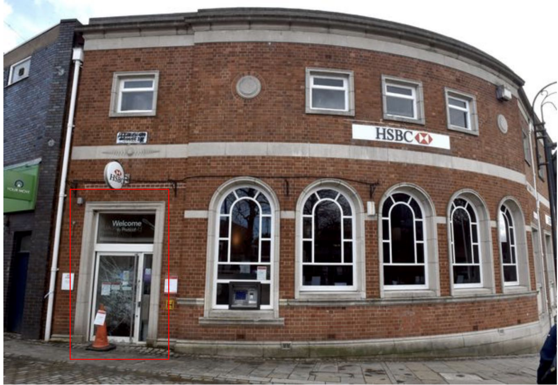
2 Eccleston Street, Prescott c.2018.
