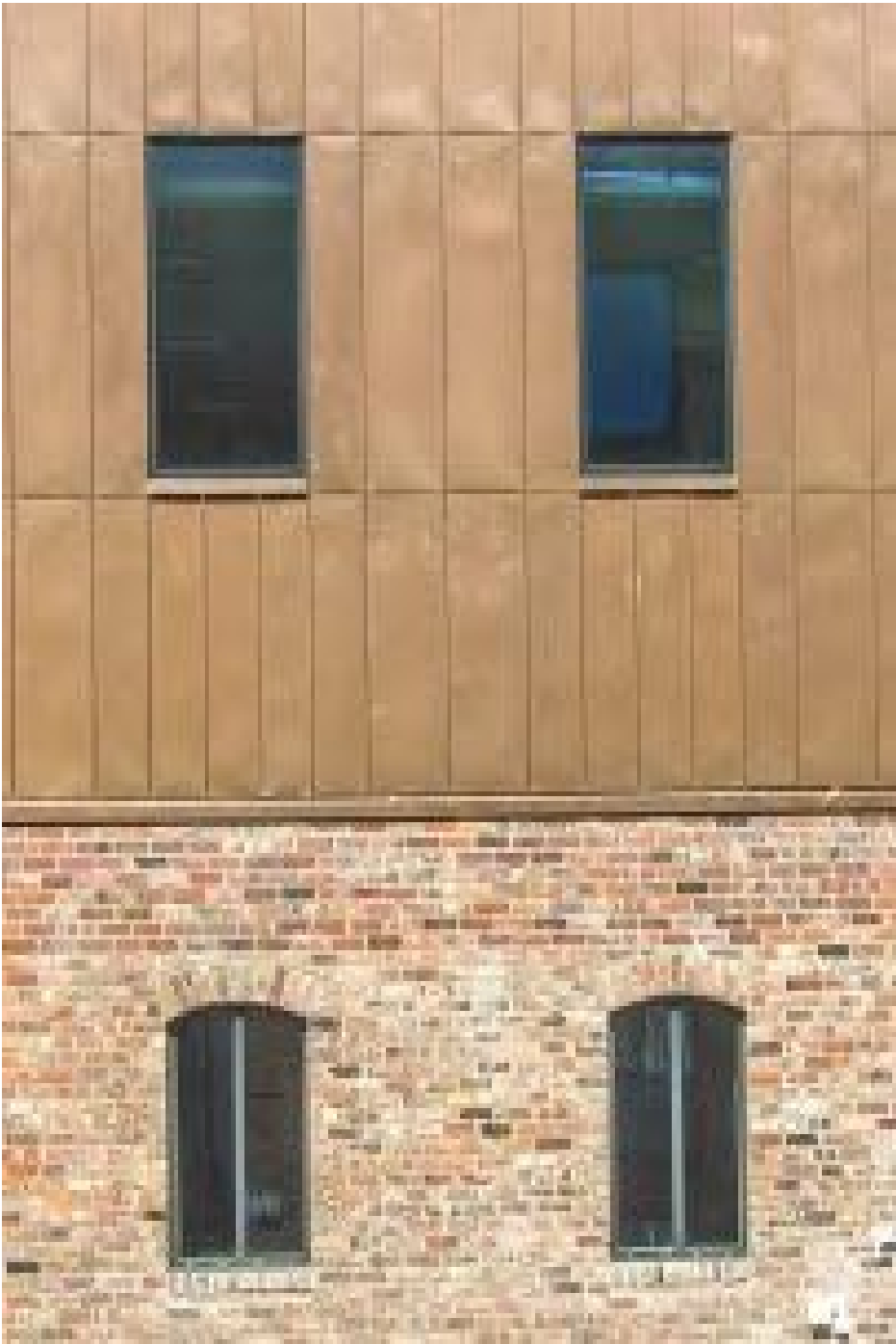
90 DUKE STREET, LIVERPOOL - KME Tecu 'Bronze' cladding. New attic storeys over historic brickwork warehouse/
