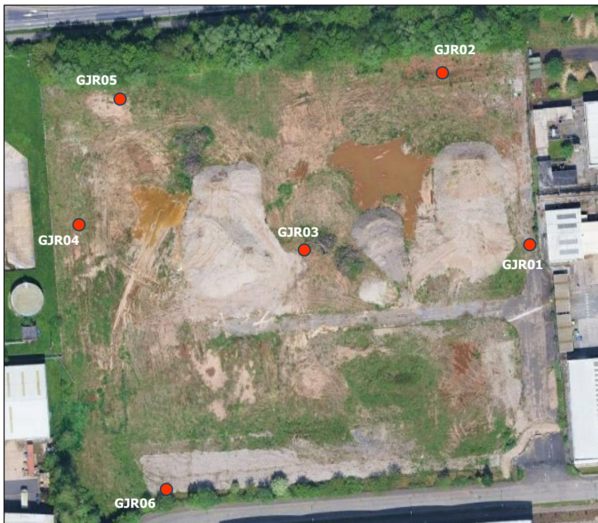
Figure 6.1 Standpipes within the Chester Formation
