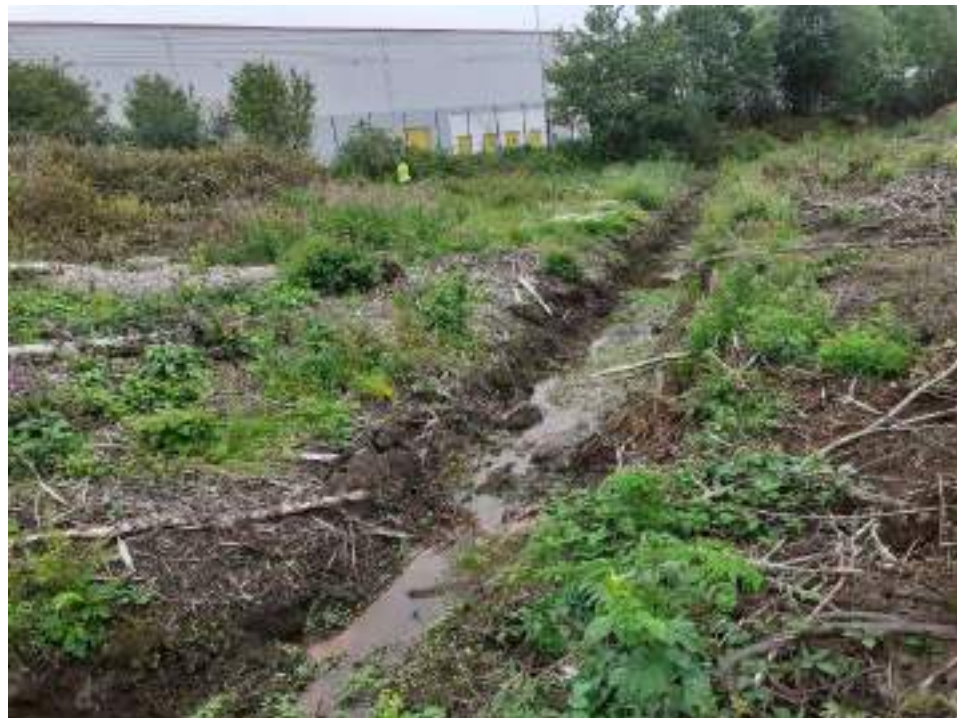
Photo 4: Offsite drainage ditch located to the northeast trending in a south easterly direction.
