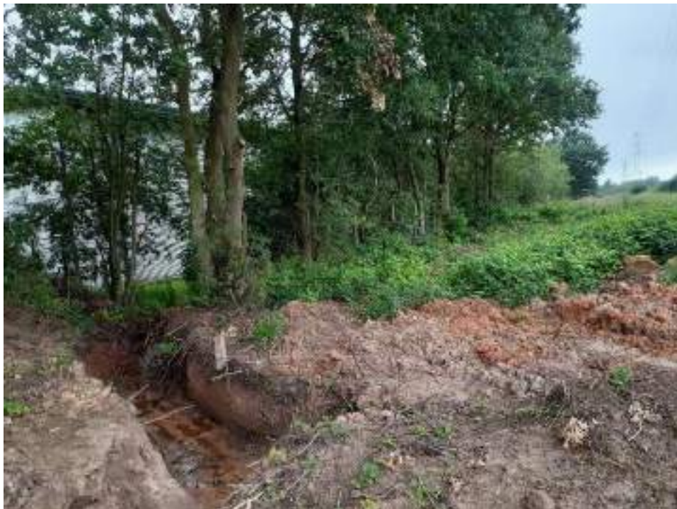
Photo 7: Modified onsite drainage channel along the southern site boundary. Water observed to be flowing in a south-westerly direction.
