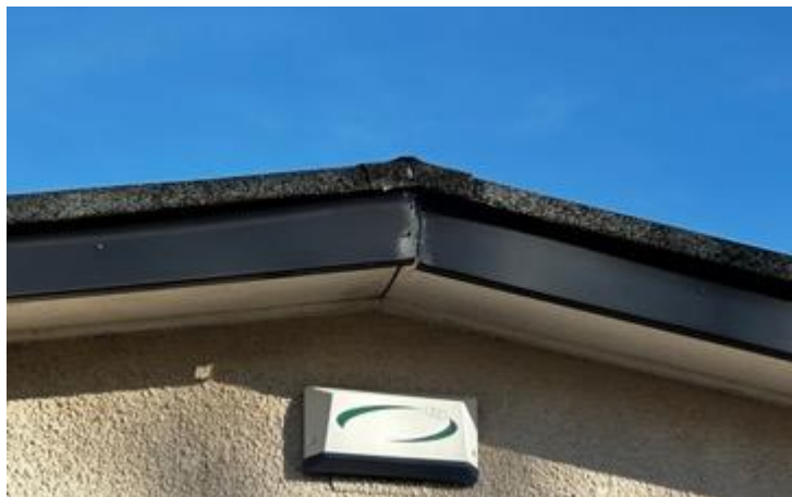
Image 5: Barge board and soffit along the southwestern elevation, intact.
