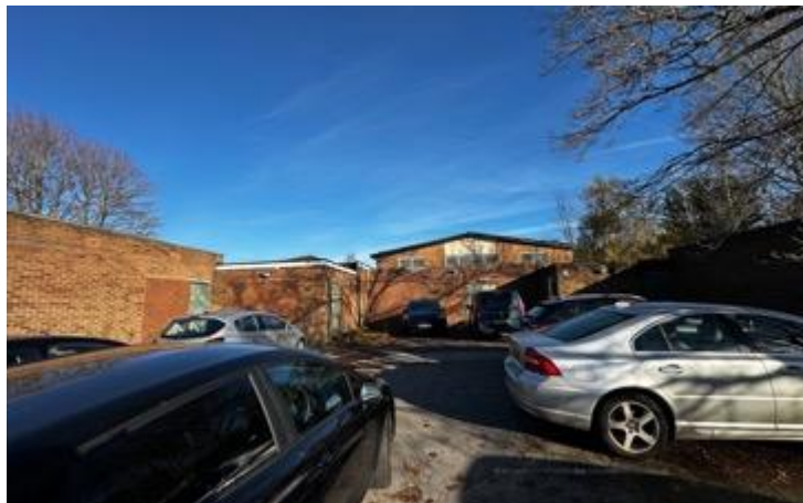
Image 3: Southwestern elevation of B1
