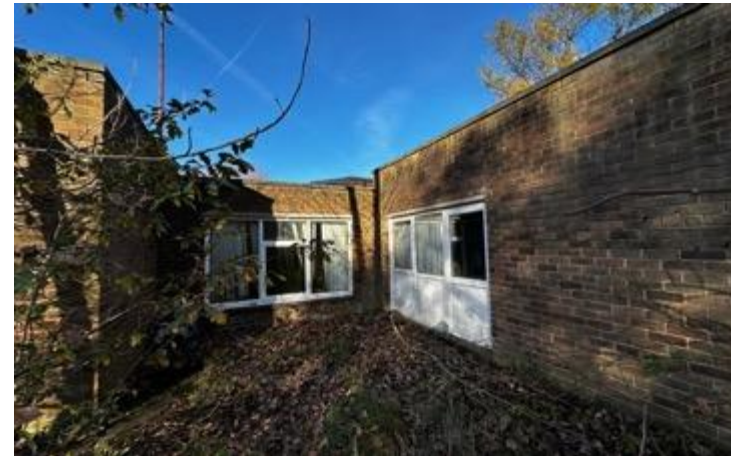
Image 2: Rear, flat roof section along the southern elevation of B1
