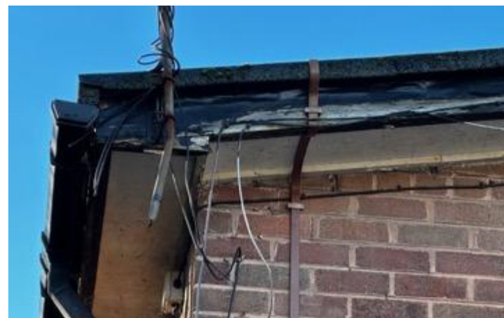
Image 8: Barge board and soffit along the northwestern elevation, intact.
