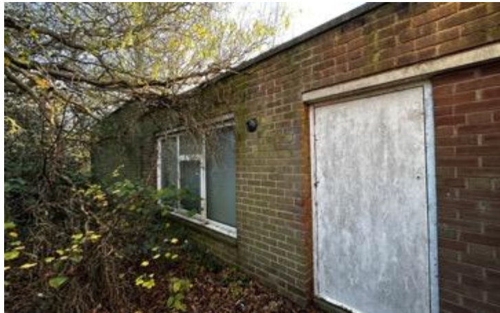
Image: 1 Rear, flat roof section along the southern elevation of B1
