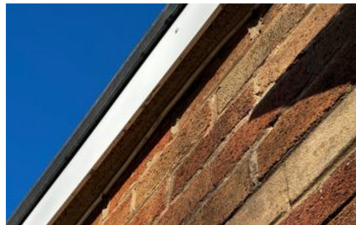
Image 6: Fascia boarding along the northwestern elevation sitting flush with the brickwork.
