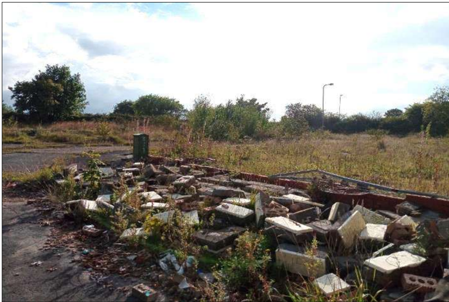
Plate 5: View of demolition material associated with the old housing estate, looking southwest
