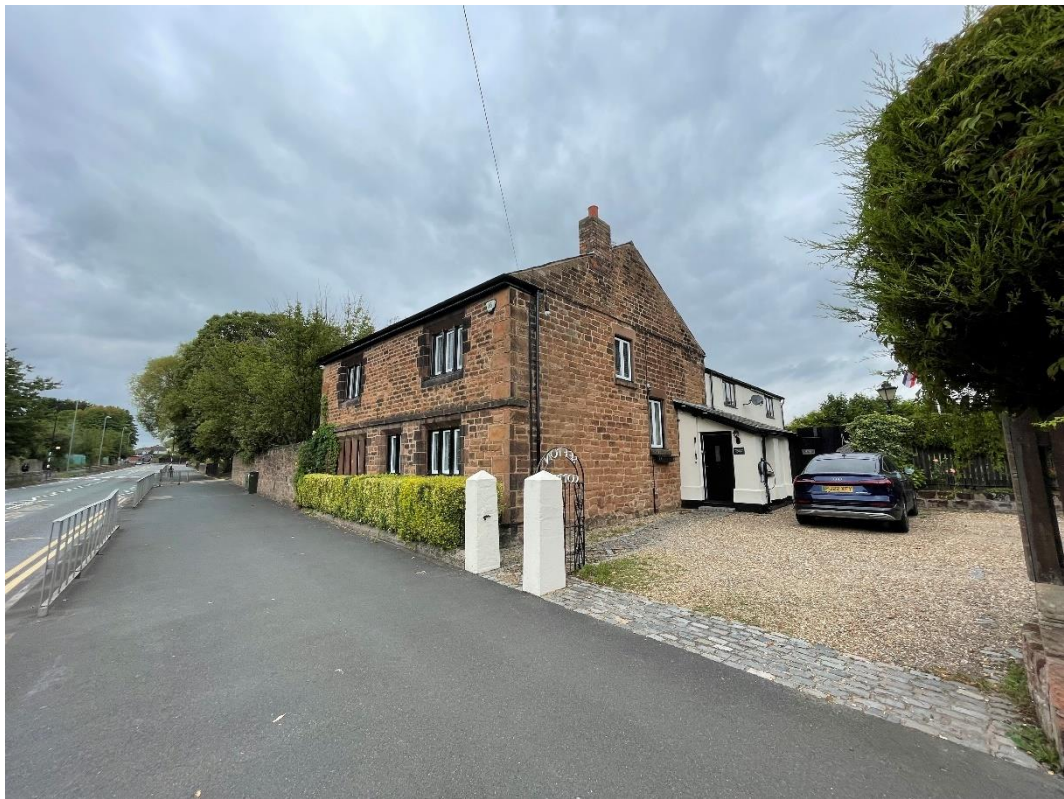
Figure 4.8: Sefton Cottage viewed from Kirkby Row
