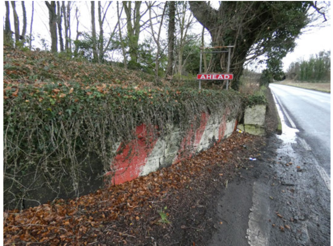
2.21 Former Entrance walls at Fox's Bank Lane. DIA
