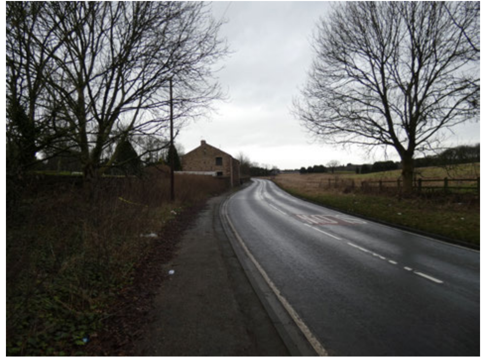
3.9 Boundary wall and Barn at Snape Gate, north of M62 (Insall)
