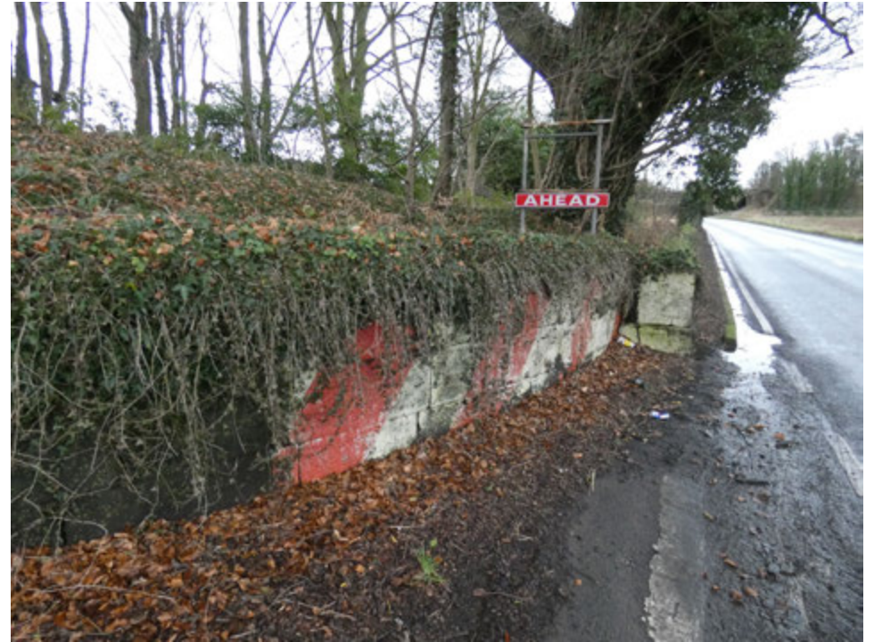
3.15 Former Entrance wall at Fox's Bank Lane. (Insalls)
