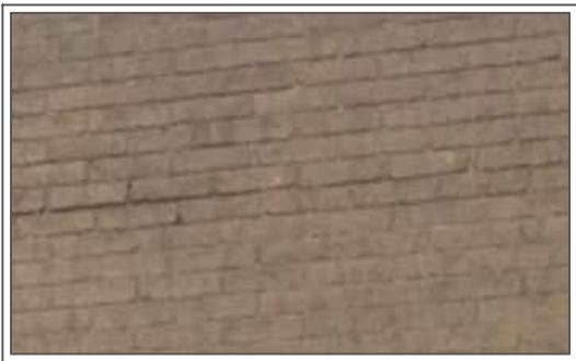
Existing brickwork to be retained and cleaned
