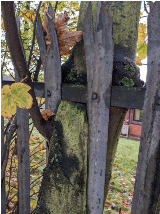
Girdling with palisade fence present on G28 & G30.
