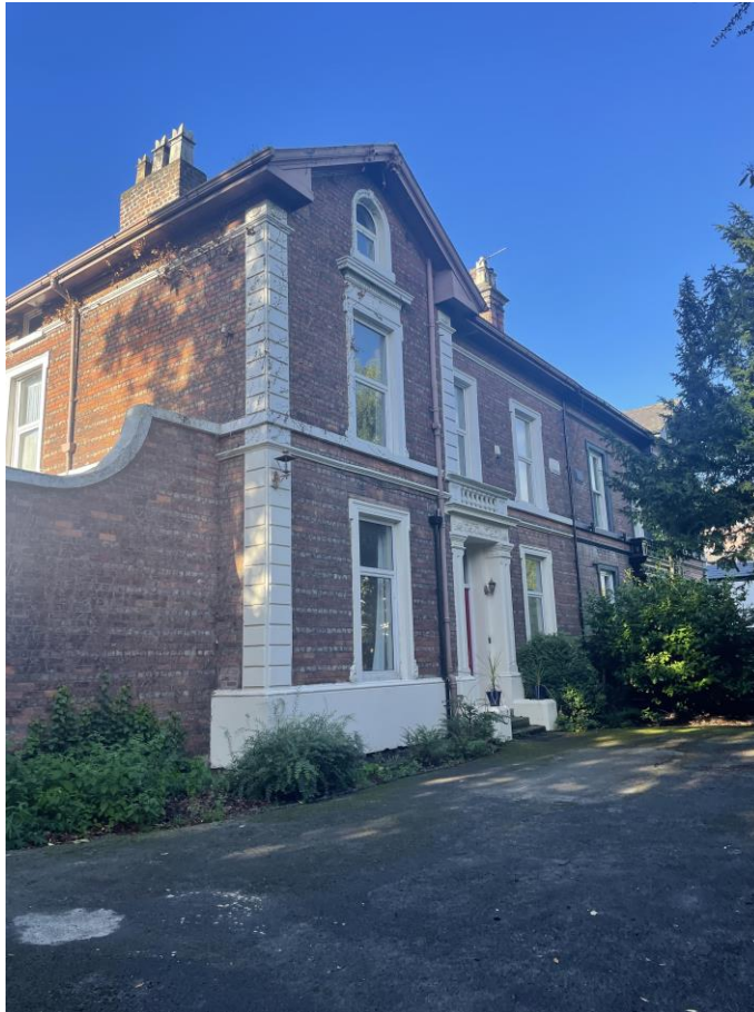
Image 2: Front elevation of No.60 St Marys Road, Liverpool.
