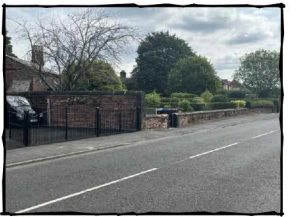
Photo 1 Street View 226 Knowsley Lane
