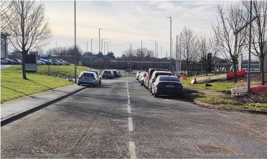
Figure 2.4 – Alchemy Way Uncontrolled Parking (looking southbound towards the A580 junction)
