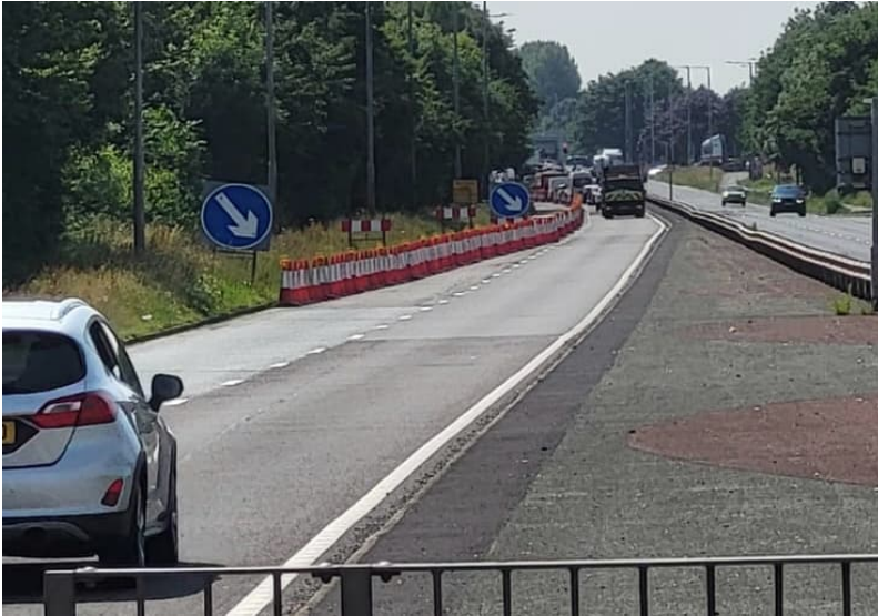
Figure 7.1 – Lane closure on the A580 Westbound, looking west from Alchemy Way
