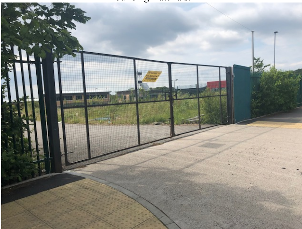
Site 2- Entrance to site from eastern boundary.
