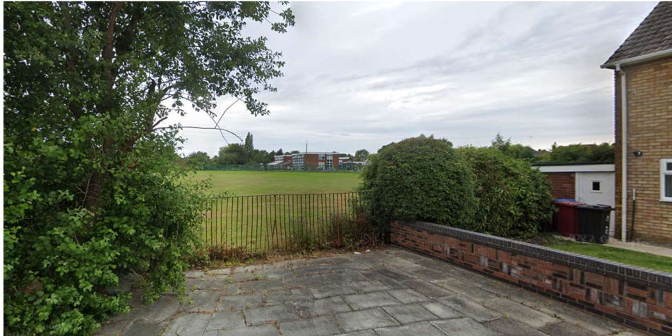
(Existing 1.5m school fencing causing security and safeguarding risk)
