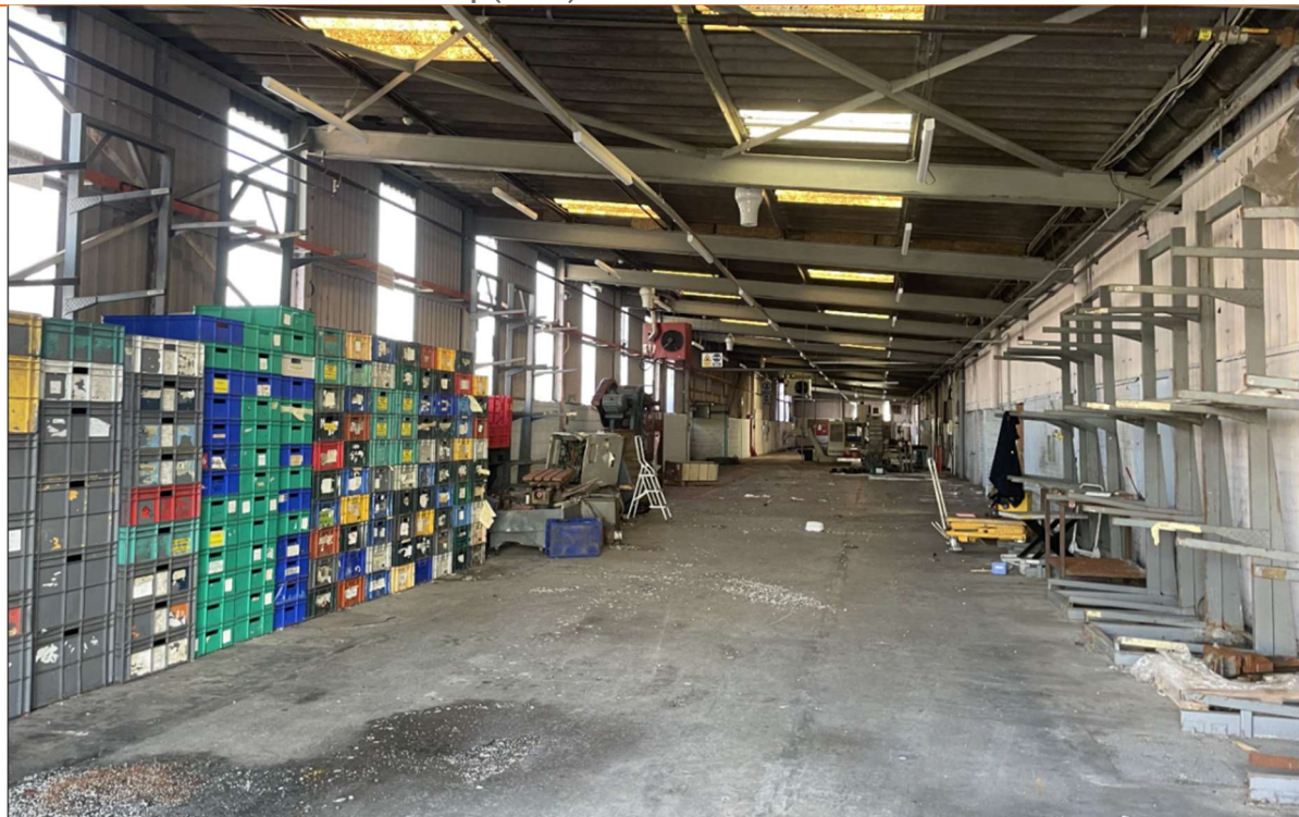
PLATE 04 Former Aluminium Shop (North)
