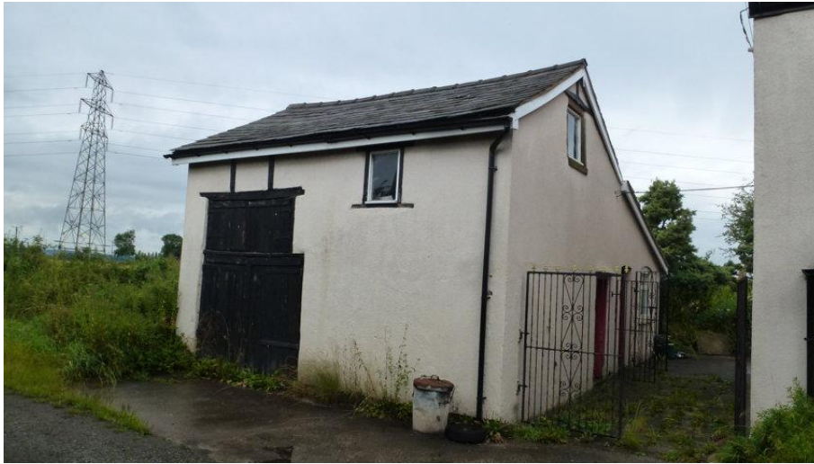
Photograph H: View of south and east facing frontages to detached workshop/garage structure.
