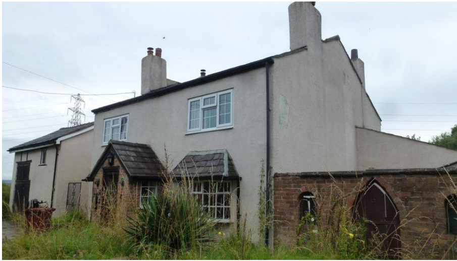
Photograph A: General View of front (south facing) and east facing gable end to residential building.
