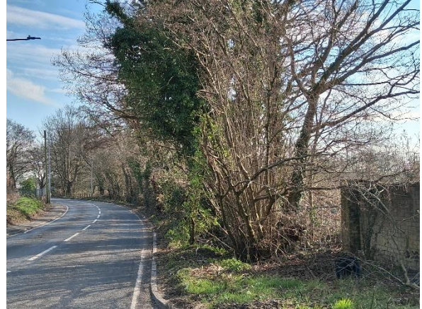
Photo 14. Trees to the eastern site boundary (Greensbridge Lane). 3 x trees to be removed at the northern end close to site entrance. (See Photos 15-17)
