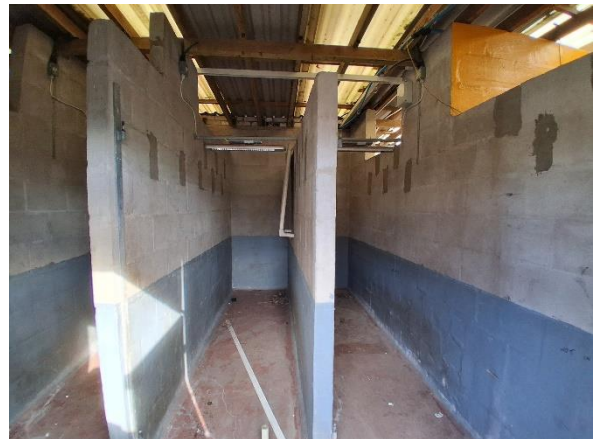
Photo 6. Interior of building 3.
