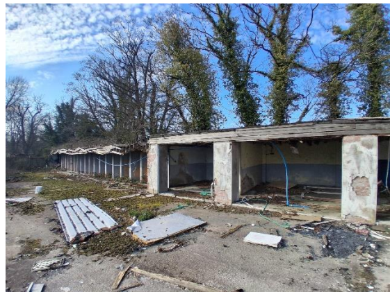
Photo 4. North-eastern end of kennels (Building.2)
