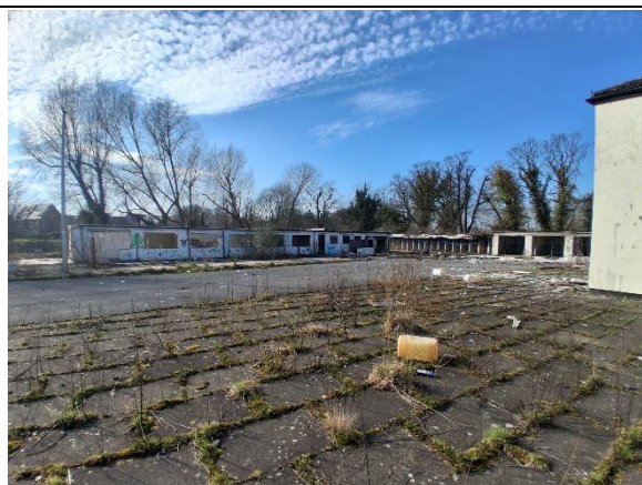
Photo 7. Main area of hardstanding (developed; sealed surface).
