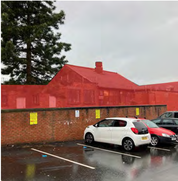
C - View from public car park.
