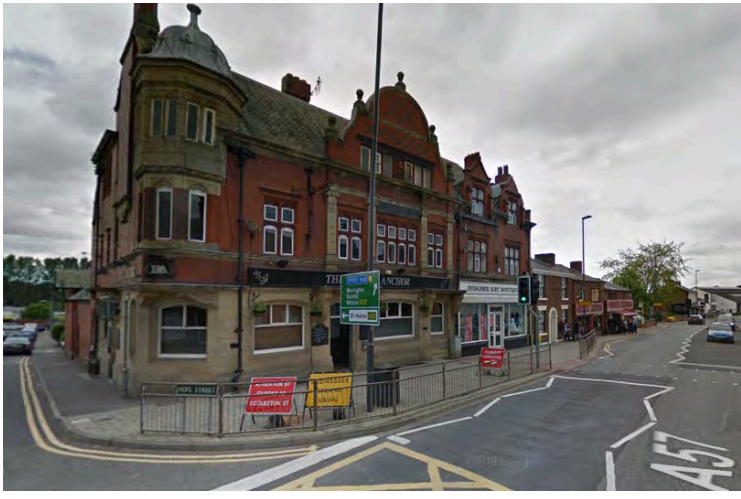
Hope & Anchor pub 'focal building' as identified in Prescot Town Centre Conservation Area Character Appraisal [May 2012]
