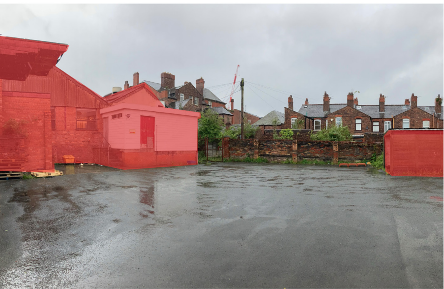
B - View from existing rear car park of both structures.
