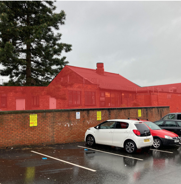
C - View from public car park.
