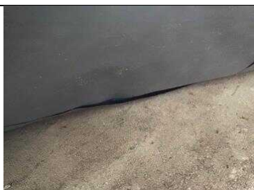
Compact substrate visible for inspection
