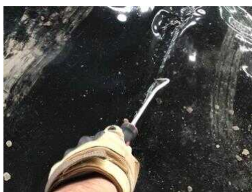
Testing to the welded lap joint to core area 2.
