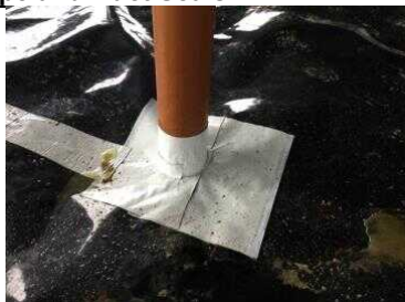
Typical pipe detail to core area 1.
