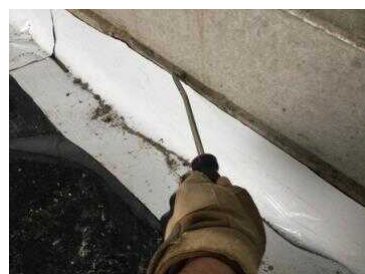
Testing along the stairwell base detail.
