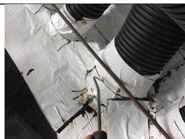
Pipe detail testing
