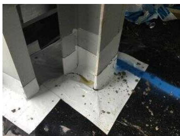
Typical stanchion detail to core area 2.
