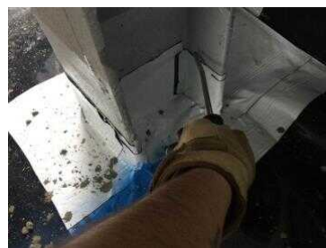
Testing to the stanchion detail within Core Area 2.
