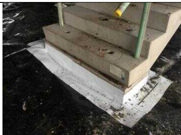
Stairwell base detailing to core area 1.
