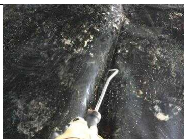
Testing to the welded lap joint to core area 1.
