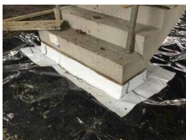
Stairwell base detailing to core area 2.
