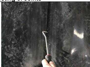
Welded lap joint testing
