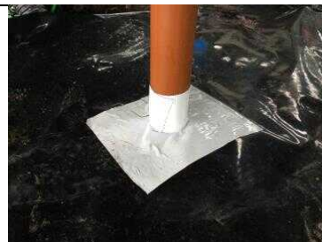
Typical pipe detail to core area 1.
