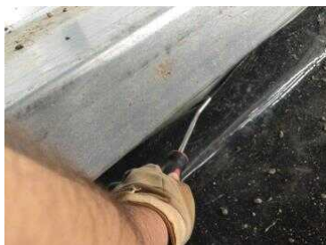
Testing to the perimeter cladding rail detail.
