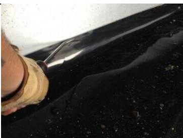
Testing along there perimeter cladding rail.
