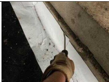
Testing to the stairwell base detail.
