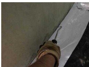
Testing along the lift shaft detail.
