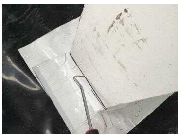
Stanchion detail testing
