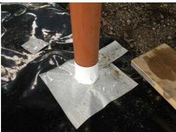
Typical pipe detail to core area 1.
