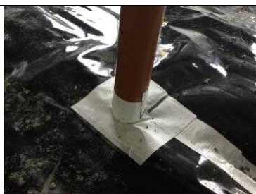
Typical pipe detail to core area 1.
