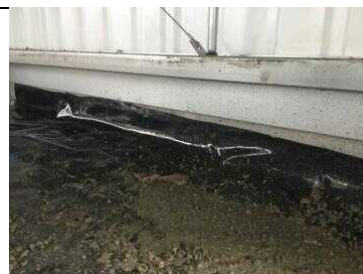
Perimeter cladding rail sealed with double sided butyl tape to Core Area 2.
