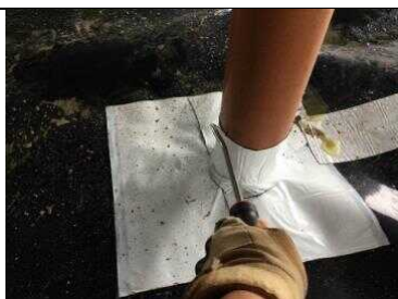
Testing to the pipe detail to core area 1.
